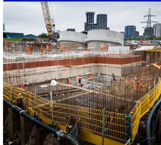
Silvertown portal/ Rotation chamber
