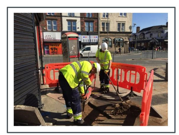
SGN's keyhole strategy aims to shift operations from conventional methods to safer keyhole technology to minimise occupation of the road network, decrease operational costs, reduce carbon emissions and limit disruption for the travelling public.
