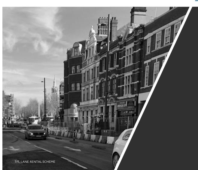
By making use of existing carriageway space and maintaining the cycle segregation, delays to cyclists were kept to a minimum, while ensuring a safer cycling environment through the road works.
