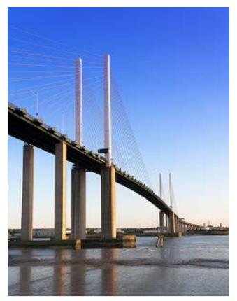
Bridges in the eastern reaches of the Thames require high clearance for shipping to pass underneath –which can mean long approach ramps
