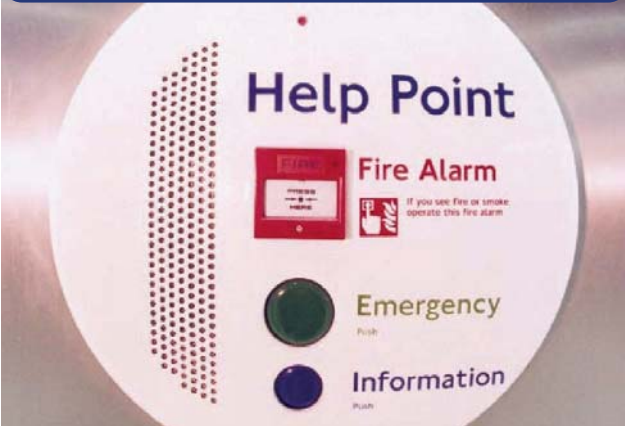
Underground platform Help Point
