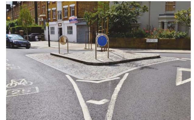
*The cobbled overrun area in this picture is in an area where motorcycles may be leant over, and could be slippery when wet. Also the white lines may guide motorcycles into the cobbled area at night, rather than around it.*
