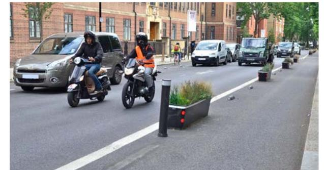
*Although more difficult to see than up-right bollards, the low level 'Zicla' separators are positioned well away from the general traffic lane and do not cause a problem for motorcyclists.*
