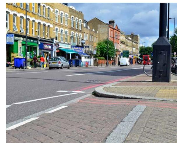
*The up ramp starts directly at the border with the main carriageway at the point where the motorcyclist will start the turning manoeuvre. There is also a change in road surface at this location.*
