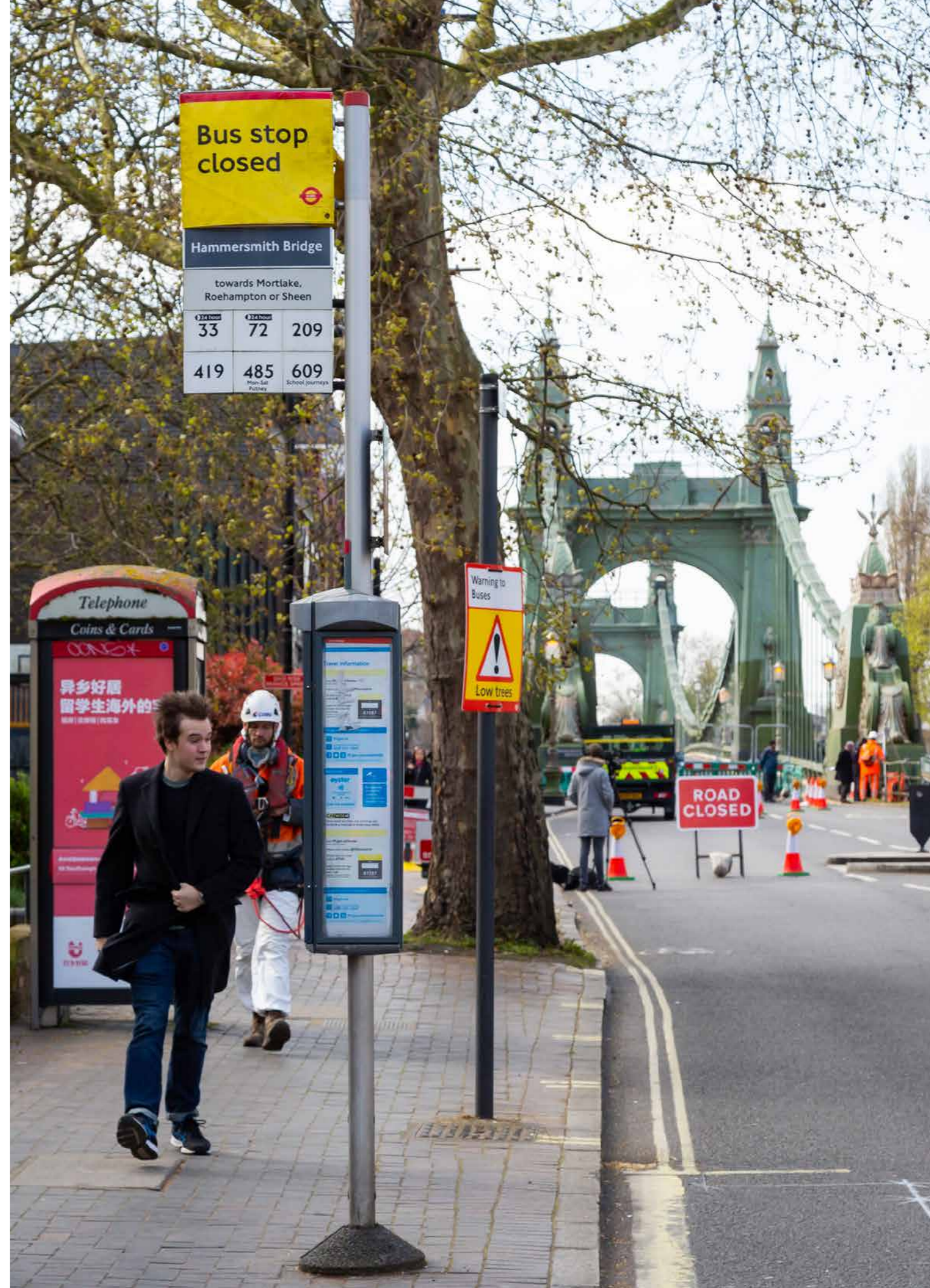
Hammersmith Bridge stabilisation work is under way
