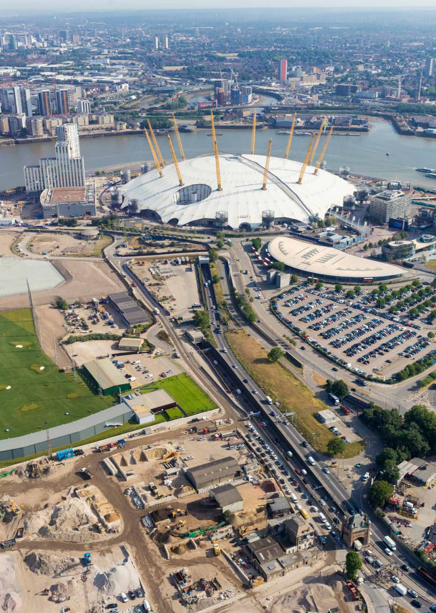
We have created a work schedule for Blackwall Tunnel
