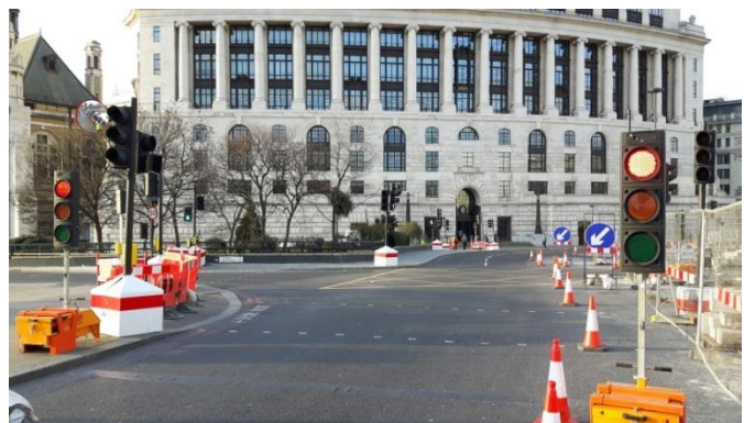
Connected portable signals in use on Blackfriars Road
