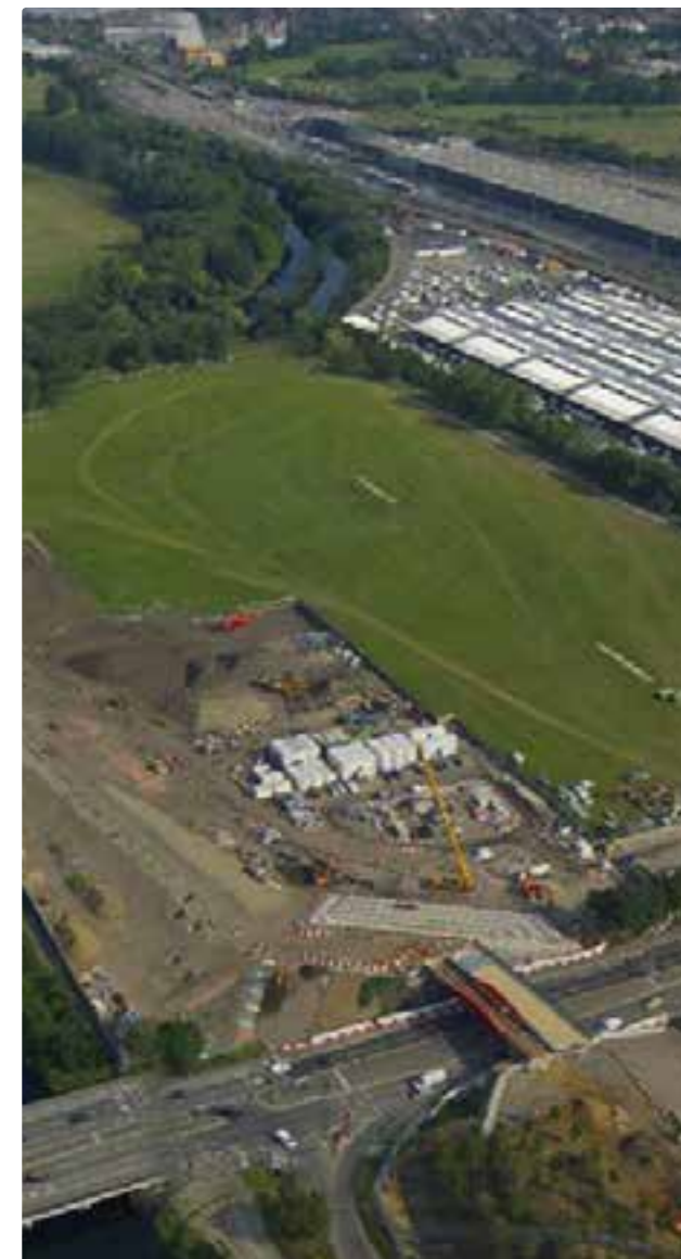
Aerial view of site under construction
