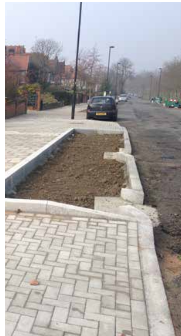
Kerb inlet and de-pave detail
