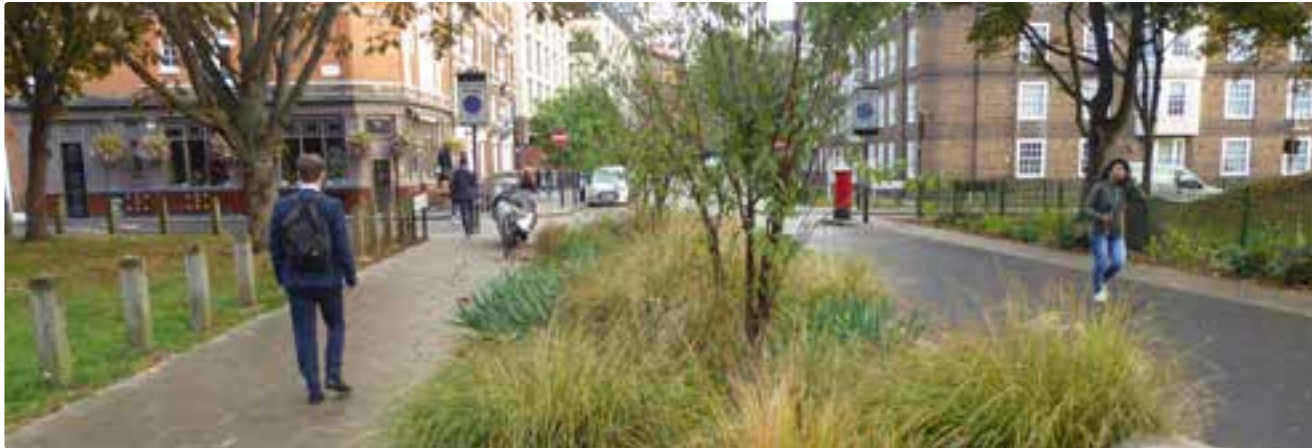
Bioretention rain garden in Vauxhall
