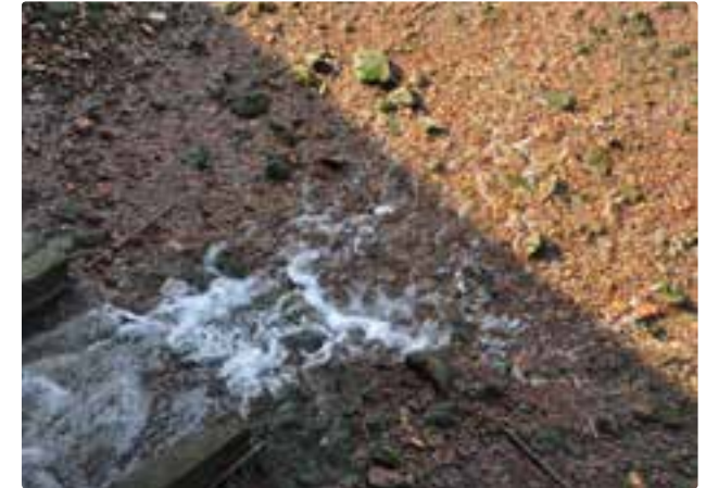
6. Surface water sewer outfall
