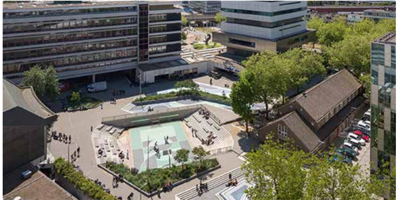
Overview of completed scheme
