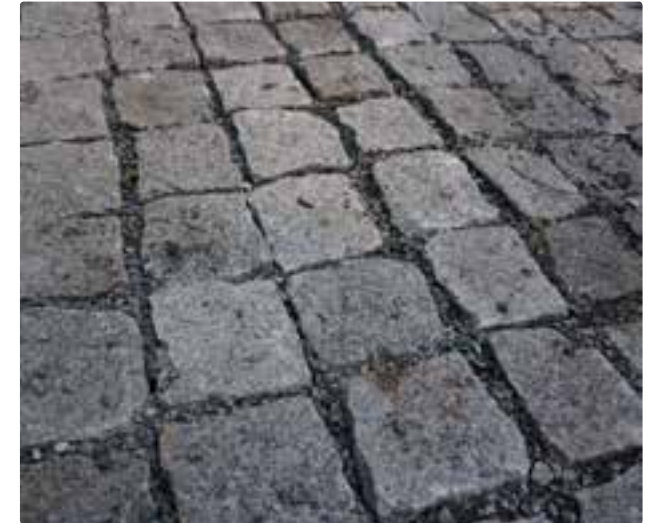
2. Grit jointed permeable paving
