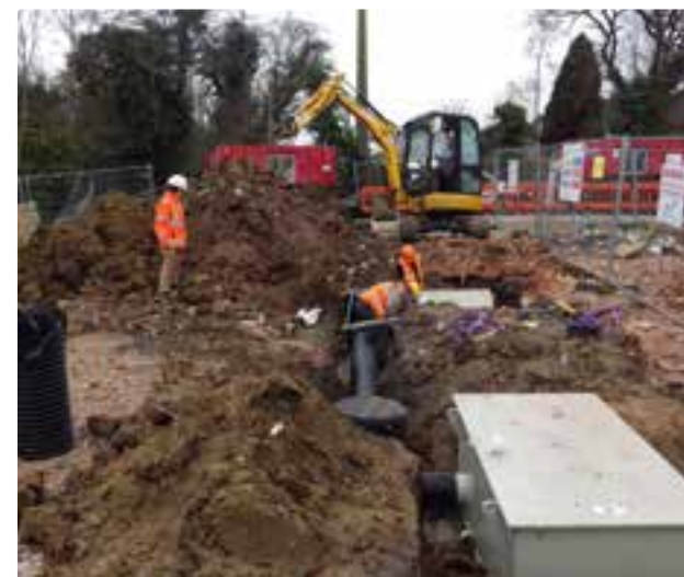
400m 2 swale under construction
