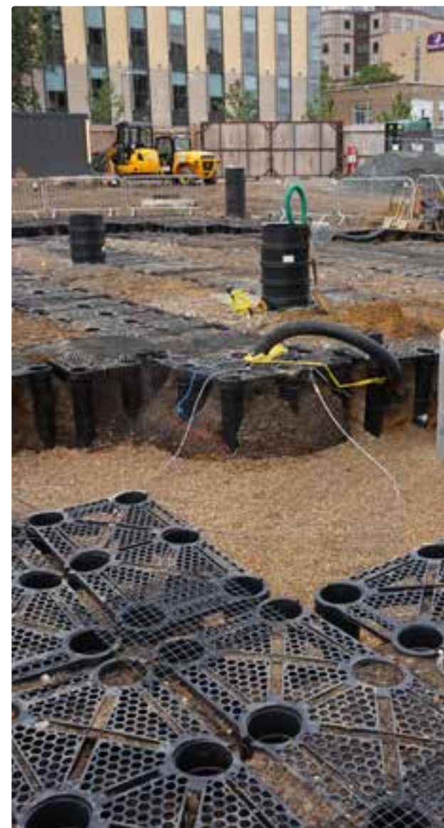
Attenuation: soil cells
