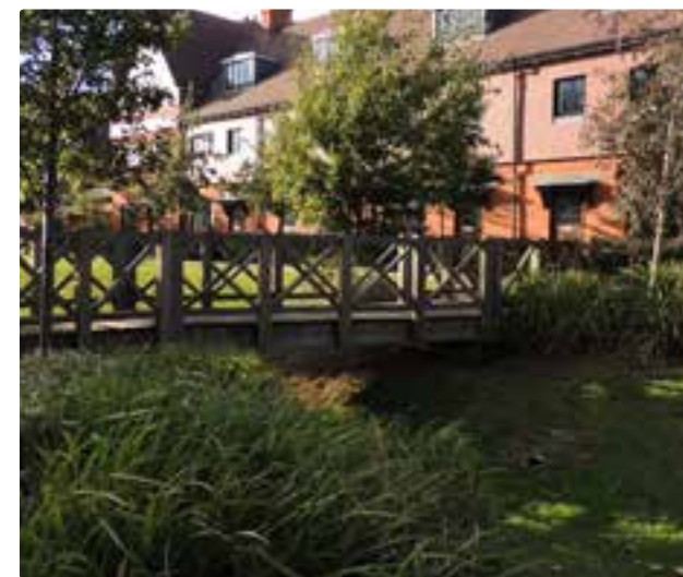
Dry swale: Upton, Northants
