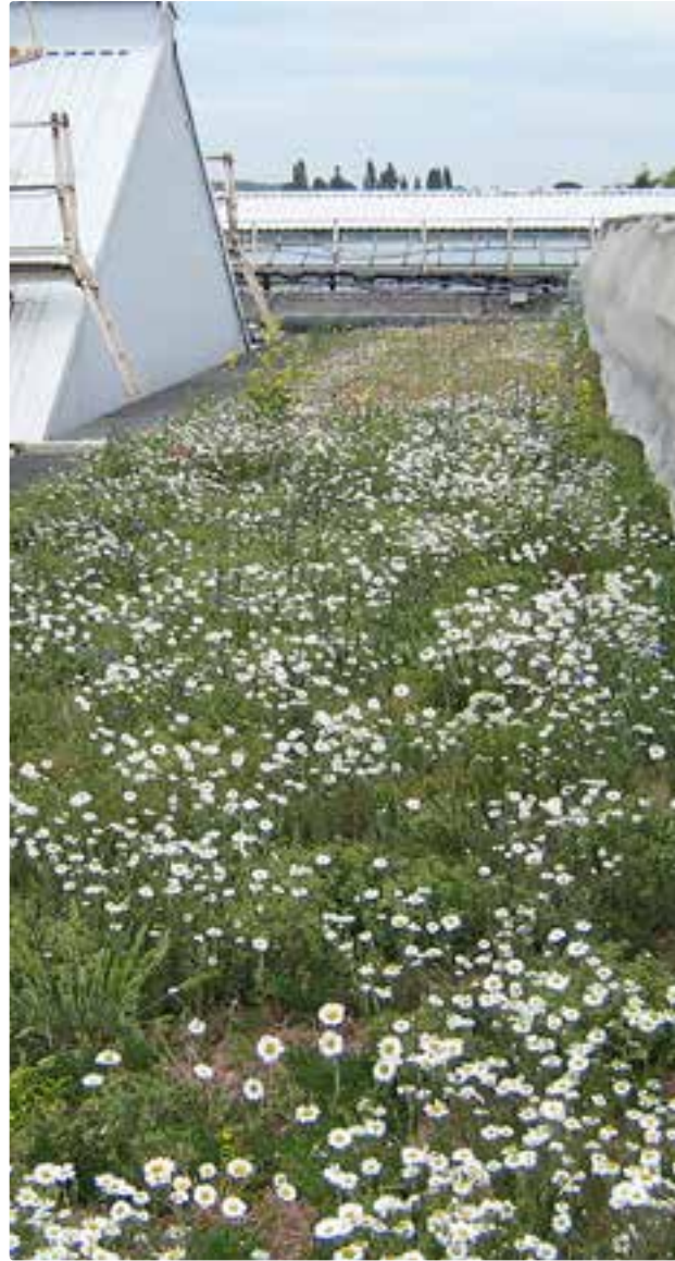
Early green roof growth within 6 months
