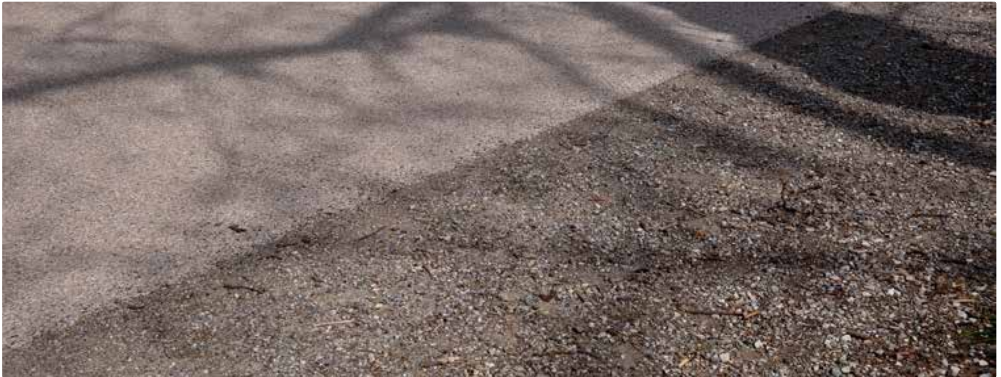
De-paving the margins of an existing pathway to increase permeability
