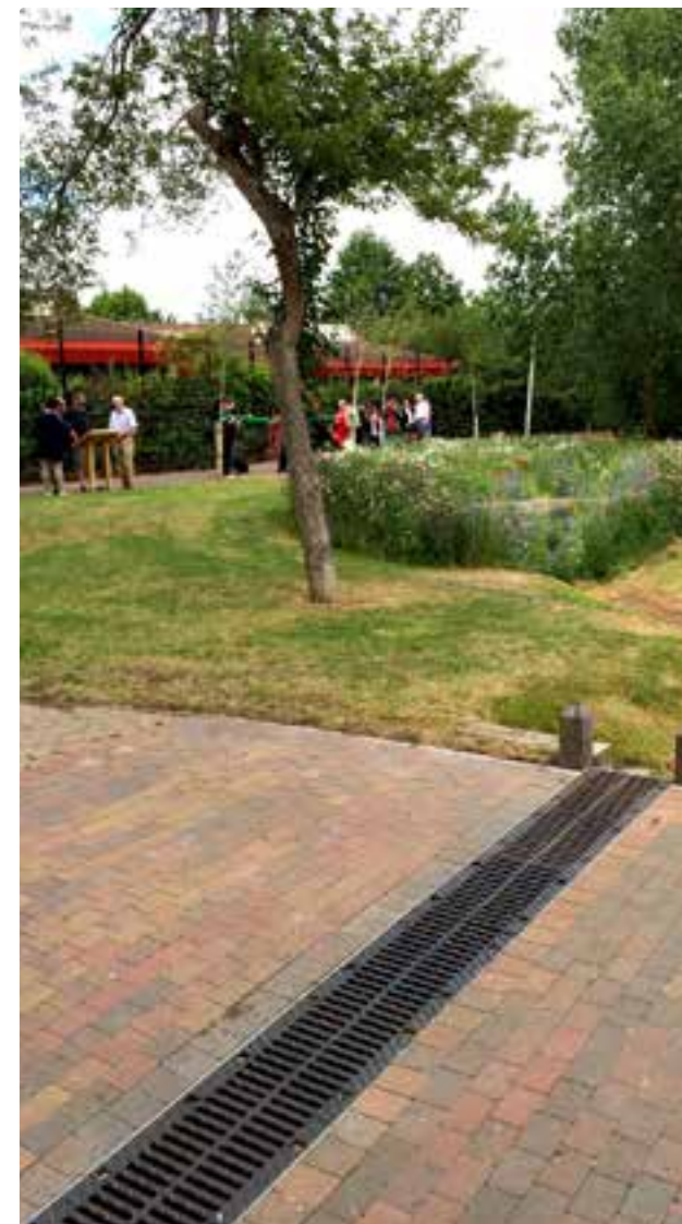
Channel outflow into swale and bioretention basin
