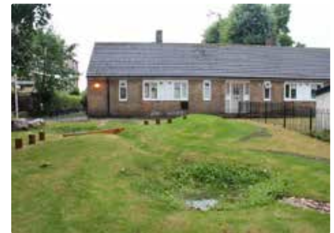
Bioretention basin outside homes
