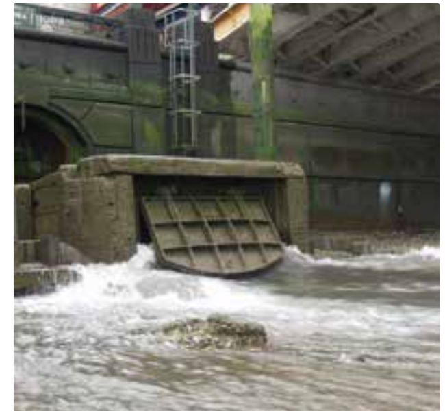
7. Combined sewer outfall
