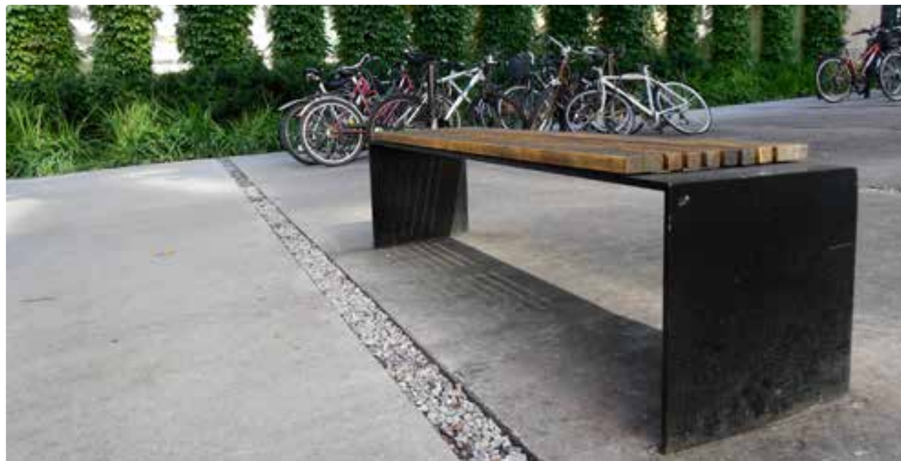
Filter drain: open gravel filled joint
