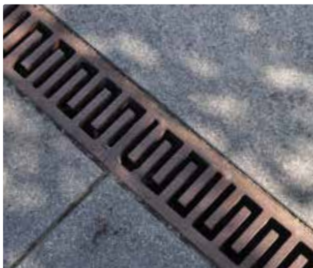
Surface water drain to root zone
