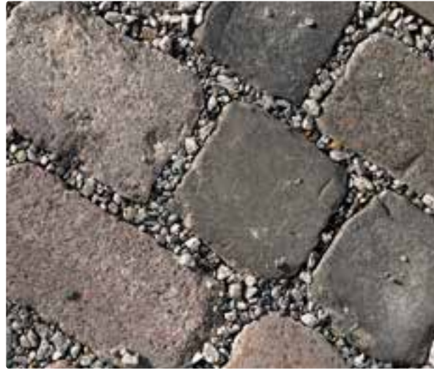
Quantity: permeable paving, grit jointing
