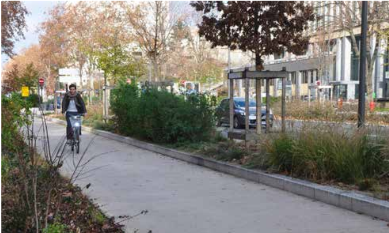
Retrofit cycleway and SuDS in Lyon
