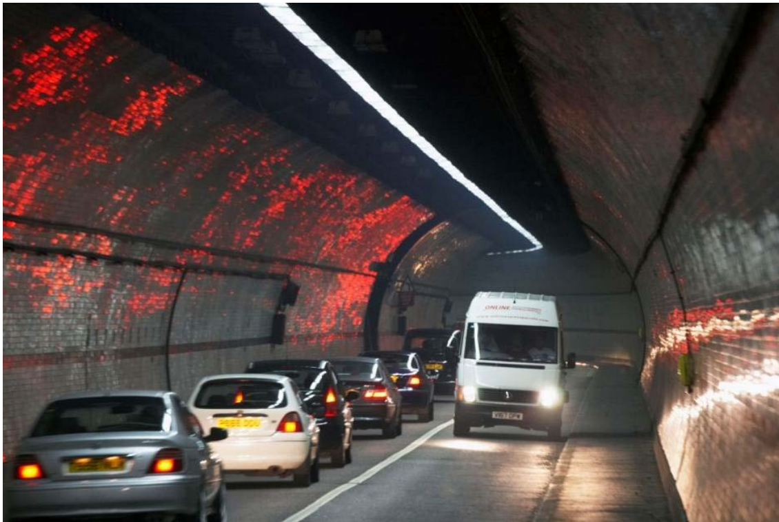
Figure 13 : Inside the Rotherhithe Tunnel, showing a bend and the narrow footway
