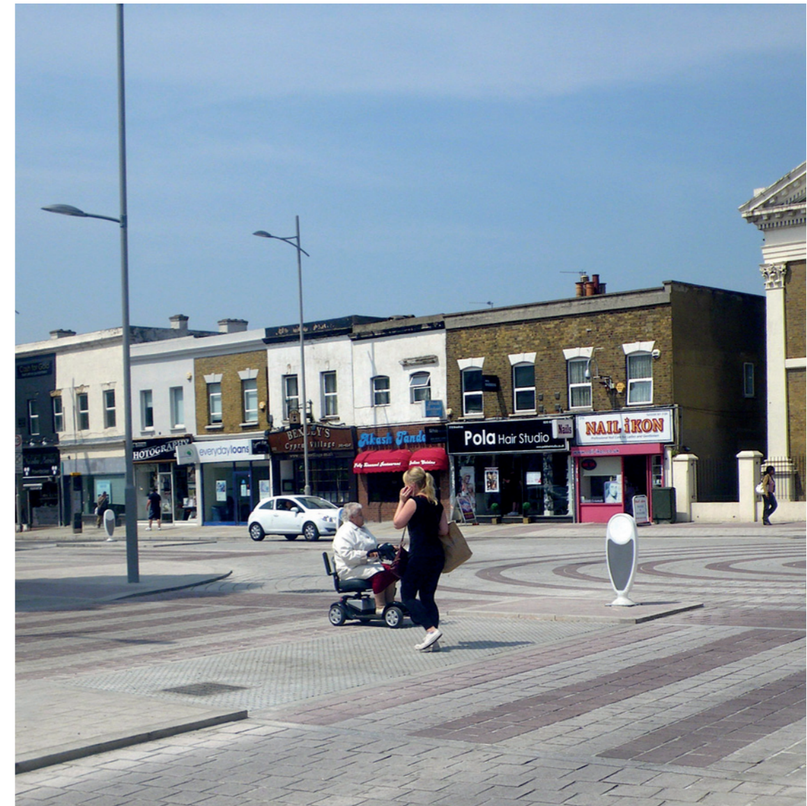
£3.5m of Local Implementation Plan Major Scheme funding delivered phase I works in Bexleyheath. These included a new roundabout on Albion Road to reduce the speed of traffic approaching Trinity Place, improved design of the junction at Albion Road symbolising a gateway to the town centre, together with the creation of a new public space outside Christ Church.
