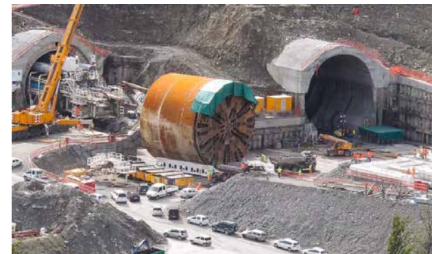
Figure 5 - Example of tunnel construction works
