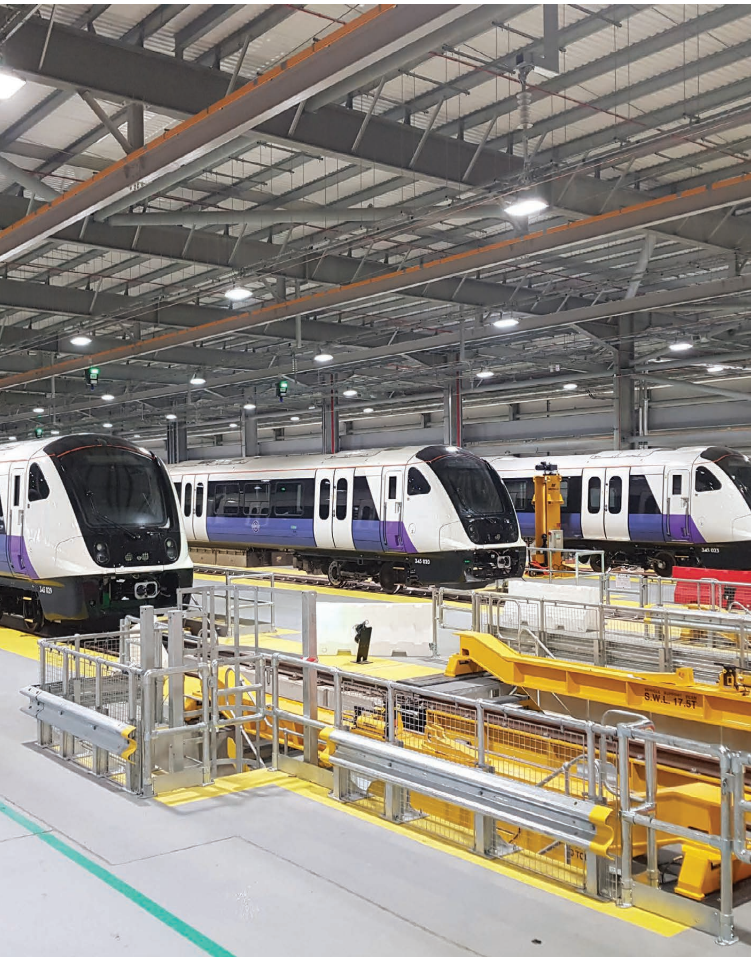
Work continues on the Elizabeth line, including ensuring step-free access is provided at stations
