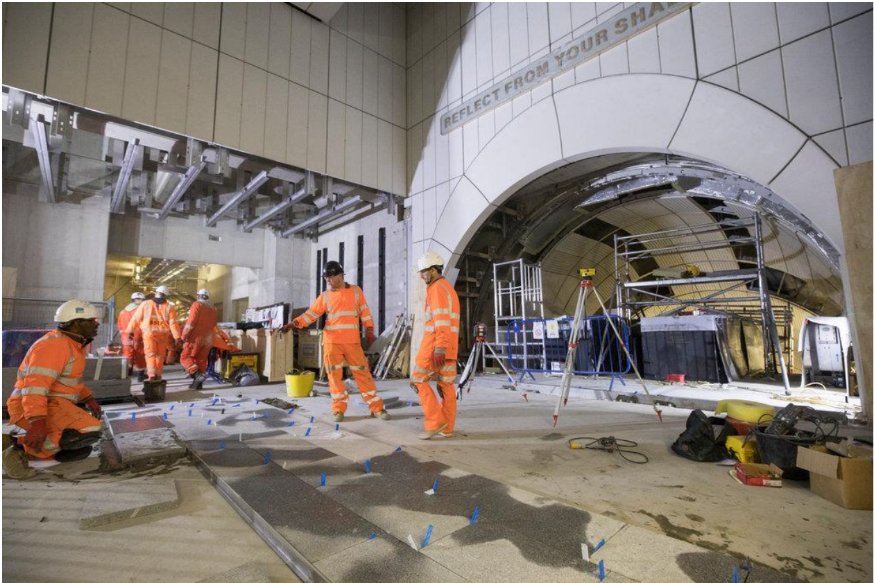
Construction Progress at Bond Street Ticket Hall
