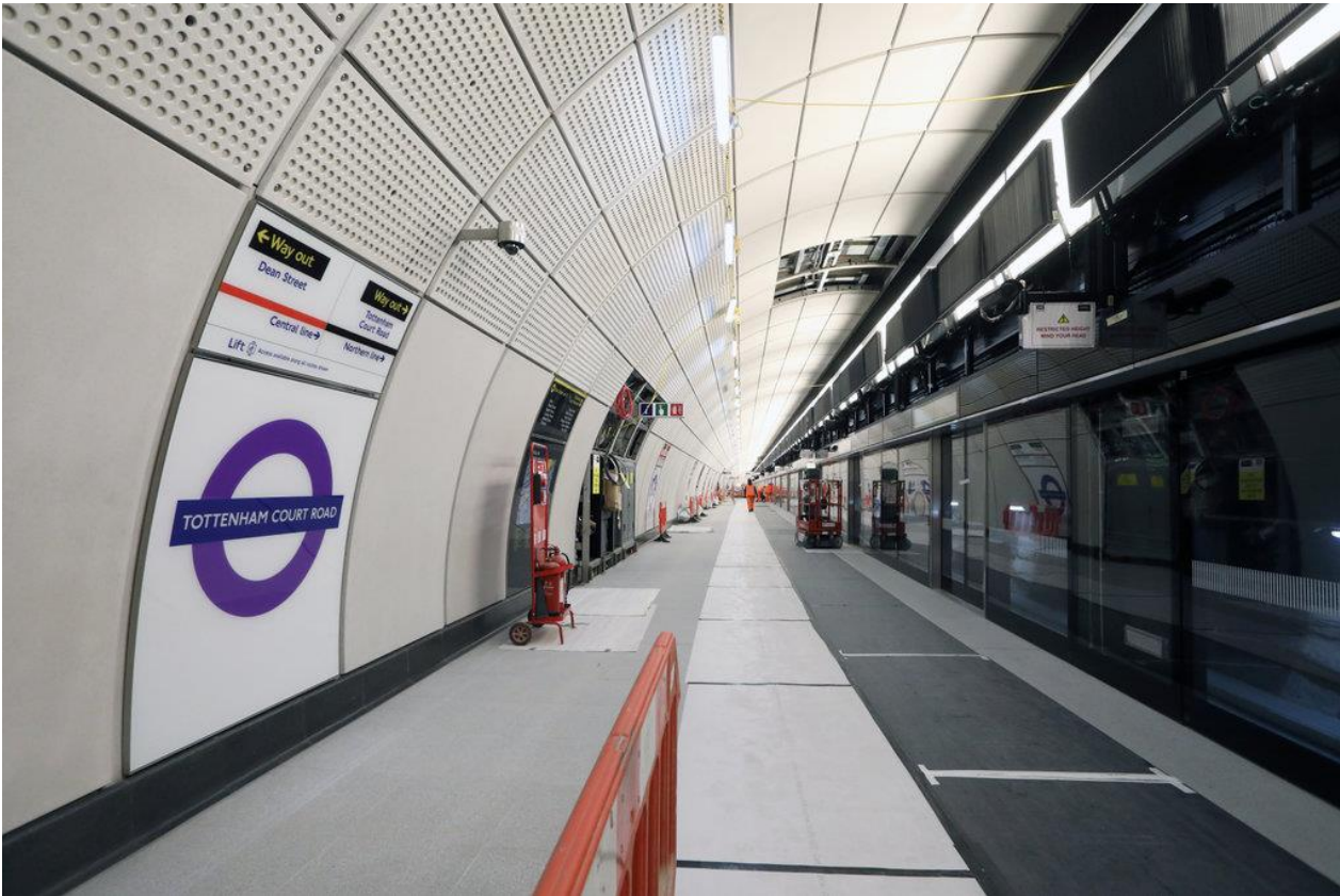
Construction Progress at Tottenham Court Road Platform
