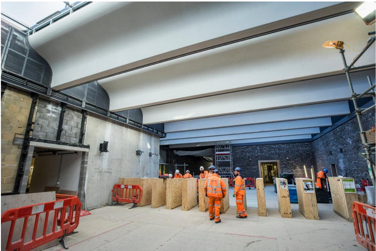
Construction Progress at Woolwich Ticket Hall
