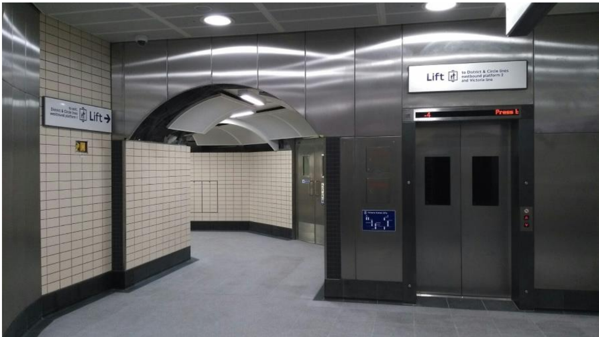
Figure 2: 1 of 7 new lifts that have made Victoria station completely step-free.
