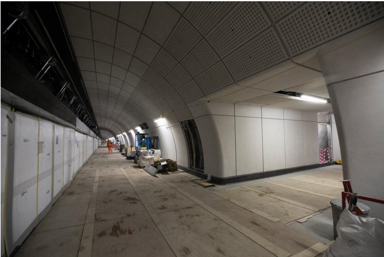
Construction Progress at Whitechapel Platform
