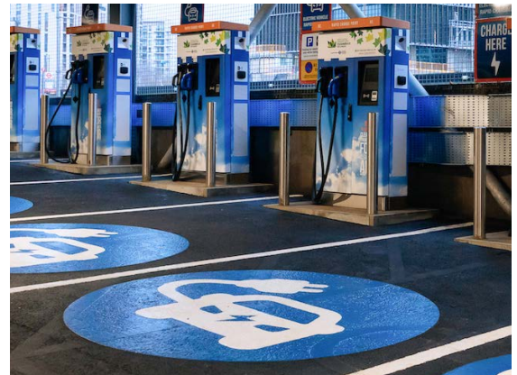
Training electric charger installers
