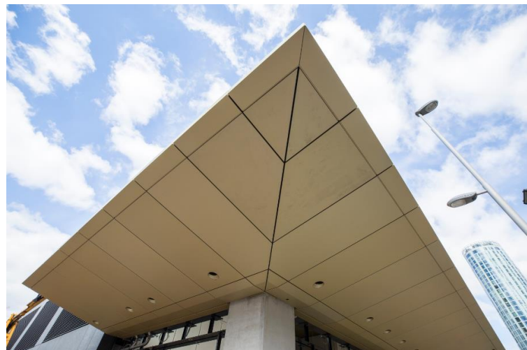
Fig. 2 The Ticket hall canopy
