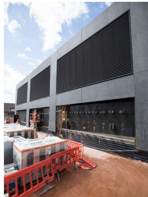
Fig.4 External cladding works
