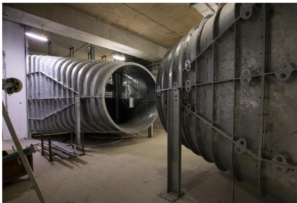
Fig.3 Fan ventilation system
