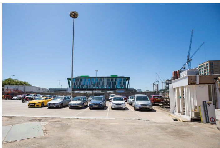
Fig. 2 One section of the newly created carpark facility
