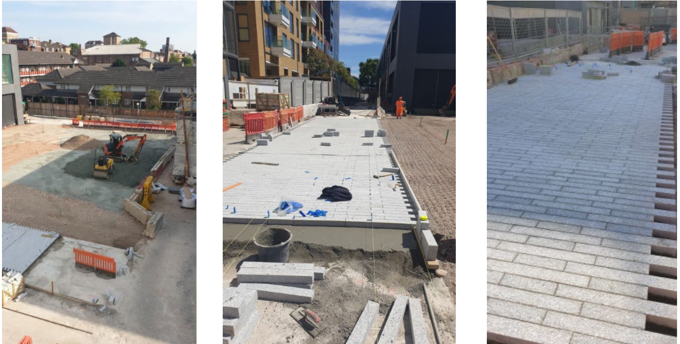
Fig.3 Hard landscaping works ongoing at 'Pascal Square' – NLE Nine Elms site
