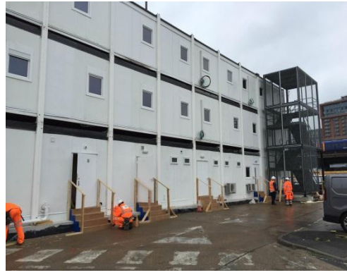
2) Installation of office cabins. Fit-out being carrying out
