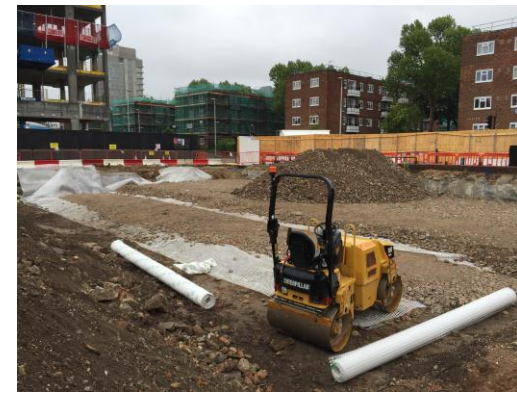
6) Piling mat construction
