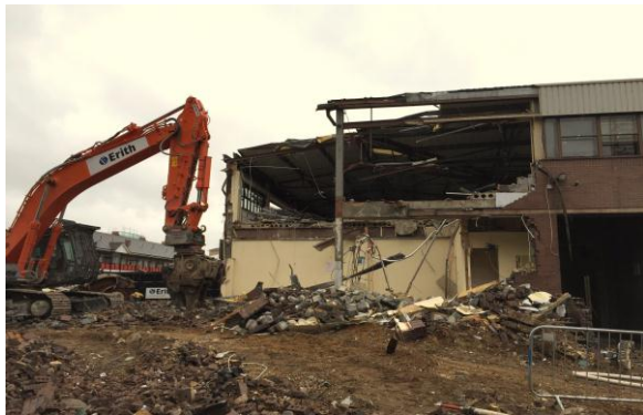
9) Covent House demolition
