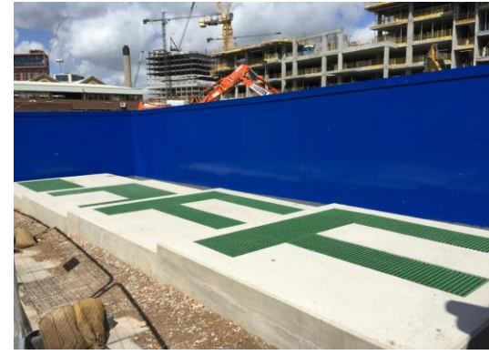
3) Substation foundations
