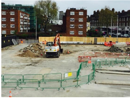
5) Tarmac removal and piling mat excavation
