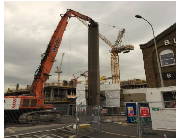
8) Boiler House demolition
