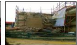
Demolition of the chimney and boiler house, Elms Elms
