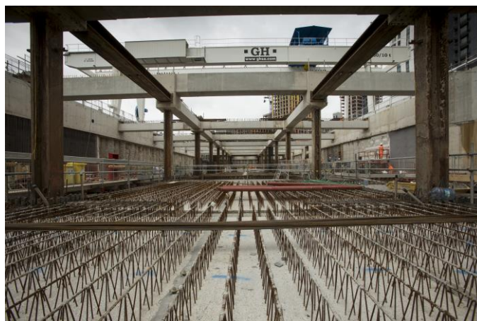
Above – installation of the pre-cast beams
