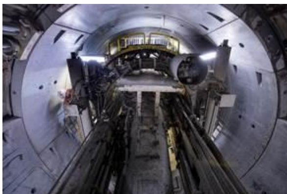
Above – a view from the back of the Tunnel Boring Machine
