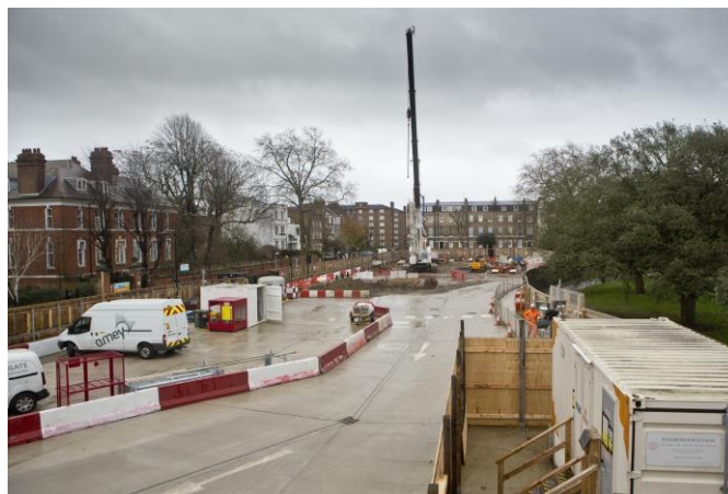
Overview of the Kennington Park site. Dec' 15
