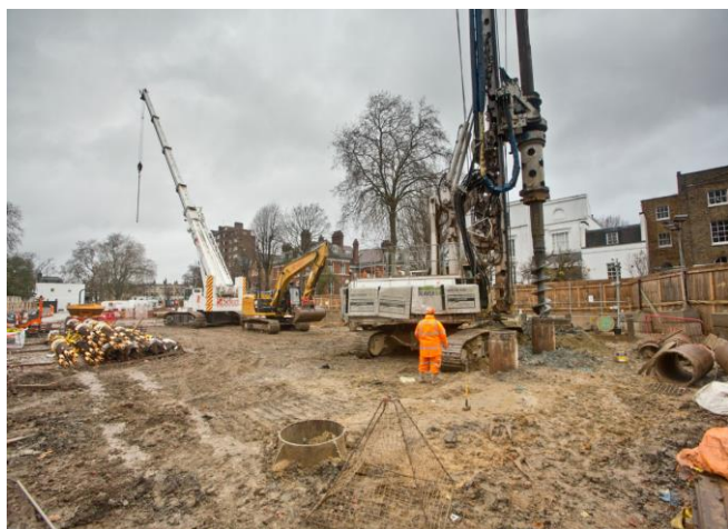
Piling Operations at Kennington Park
