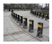
**Inset** – steel plate set into a concrete base e.g. shallower dig required.
