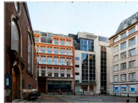
8 | Looking out of Abchurch Yard towards the application site
