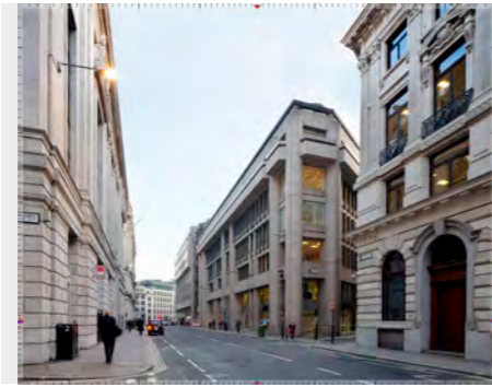
2 | Looking south-east along King William Street from its junction with Abchurch Lane
