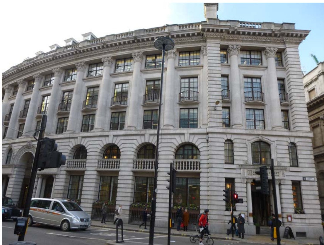
Photo 1: General view of 1-6 Lombard Street
