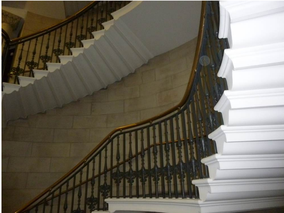
Photo 3: Cantilevered main stair
