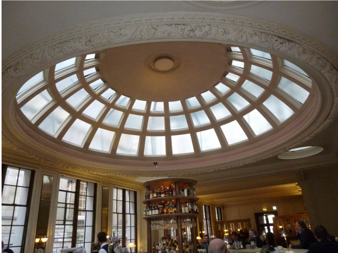
Photo 2: Dome of restaurant with decorative plaster enrichment
