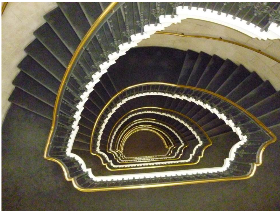
Photo 4: View through well of stone cantilevered stair.
