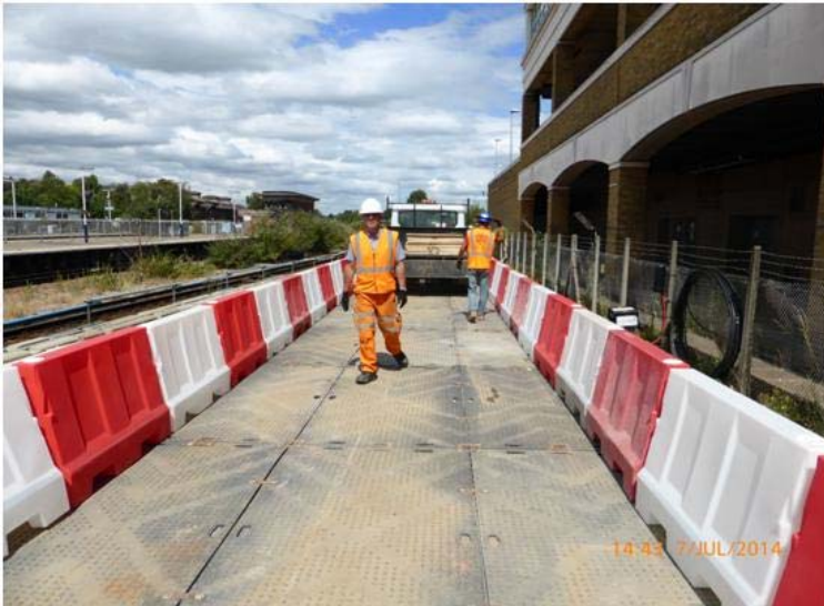
Platform track slab laying at Wimbledon station
