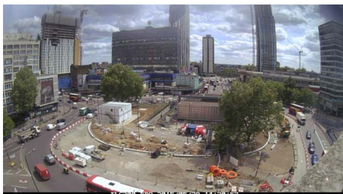
Time lapse captured on 28 May 2015 for the northern roundabout works
