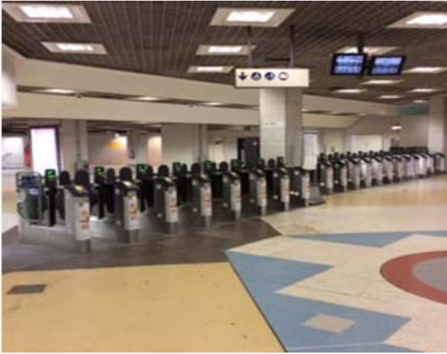
Relocated Liverpool Street station gate line
