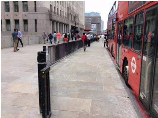
London Bridge footway repaving scheme
