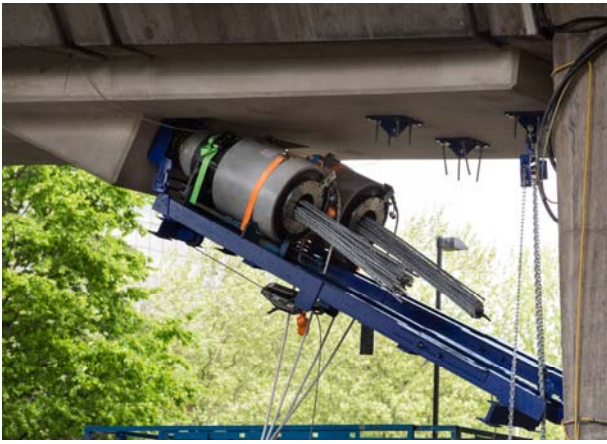
Tensioning of the internal long tendons
