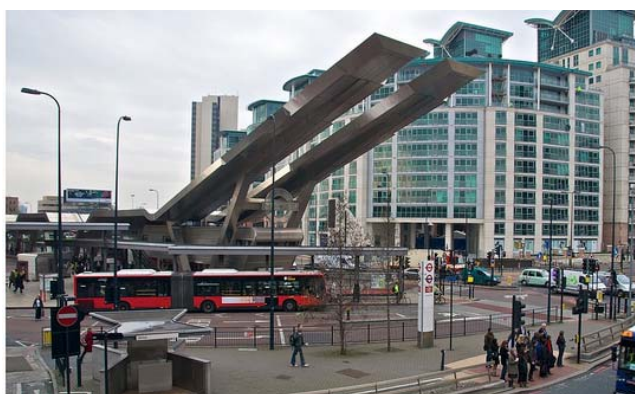
Vauxhall station entrance and bus stops
