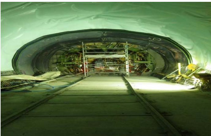
Victoria Station Upgrade junction waterproofing
