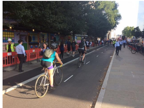
Cycle lane narrowed to allow footway to be temporarily widened
