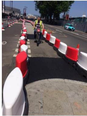
Segregated island converted to a temporary cycle lane and the permanent cycle lane converted to a footway CS7
