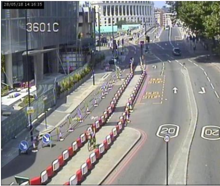
Segregated island converted to a temporary cycle lane and the permanent cycle lane converted to a footway CS7
