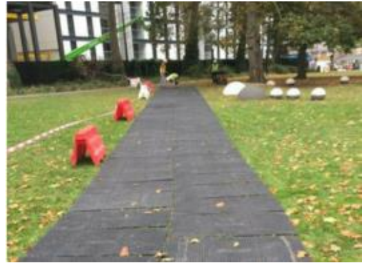
Recreational land converted to a temporary cycle lane with matting system to continue CS7
