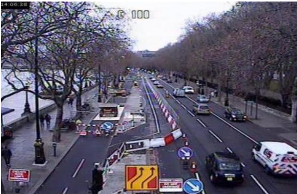
Carriageway lane converted to a temporary cycle lane widened
