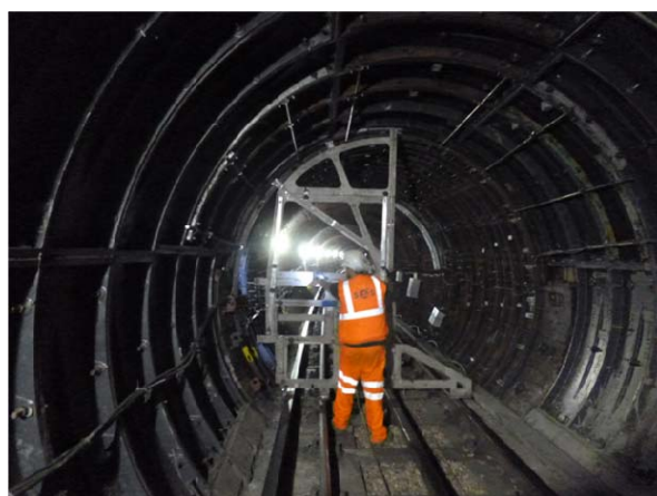
Gauging survey following ring installation
