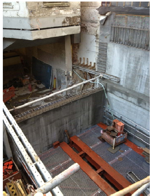
Substation silo steelwork-lower platform
