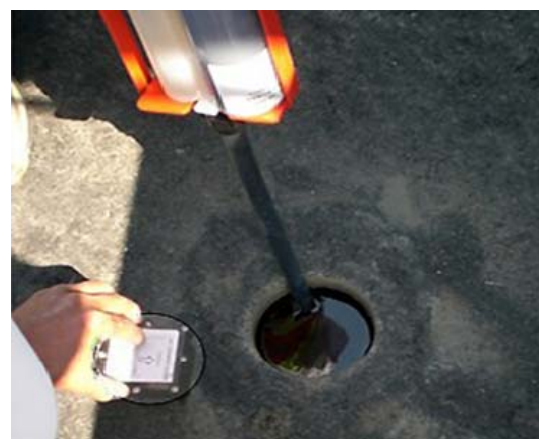
Protective sealant applied
