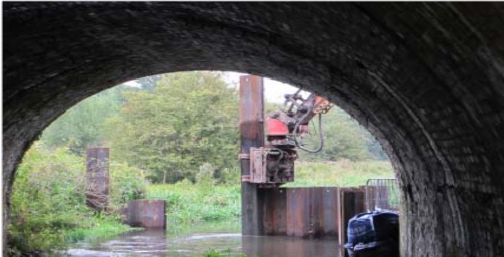
Diversion of River Gade for bridge scour works
