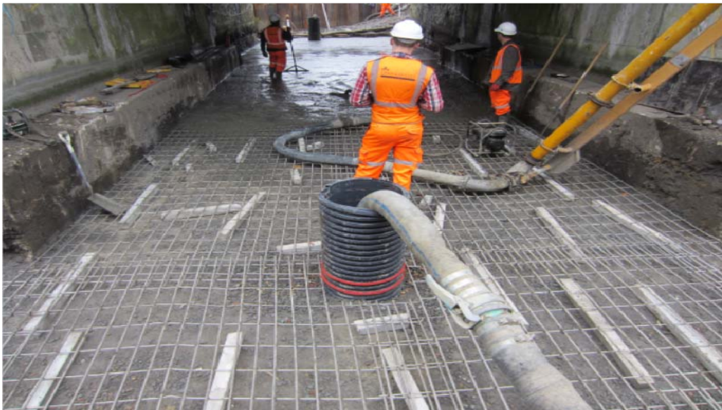
Installation of reinforcement bars before concrete pour
