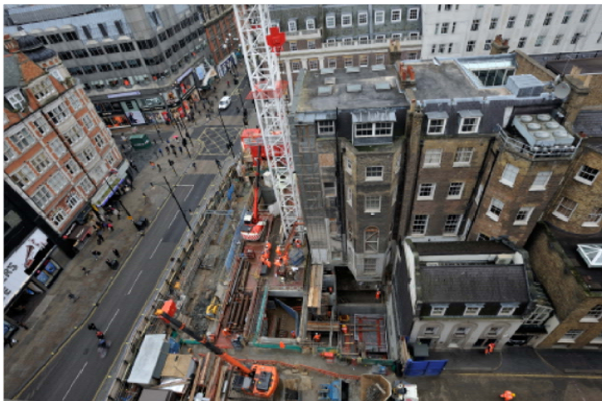
View over site
