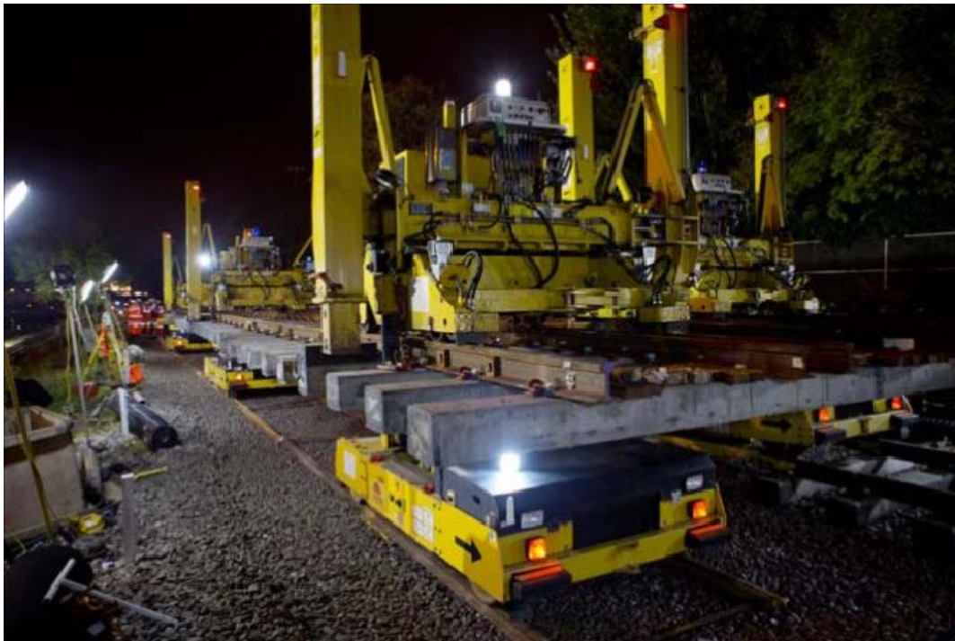
The remodelling and installation of a critical section of the network at Acton Town
