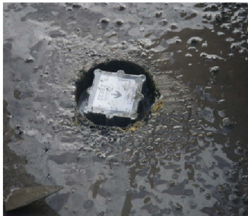
A magnetometer in the carriageway
