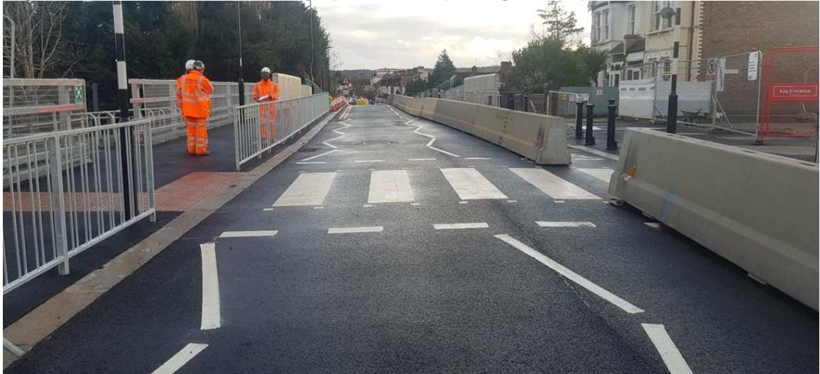
Figure 2 Exterior view of the new entrance at West Hampstead station
