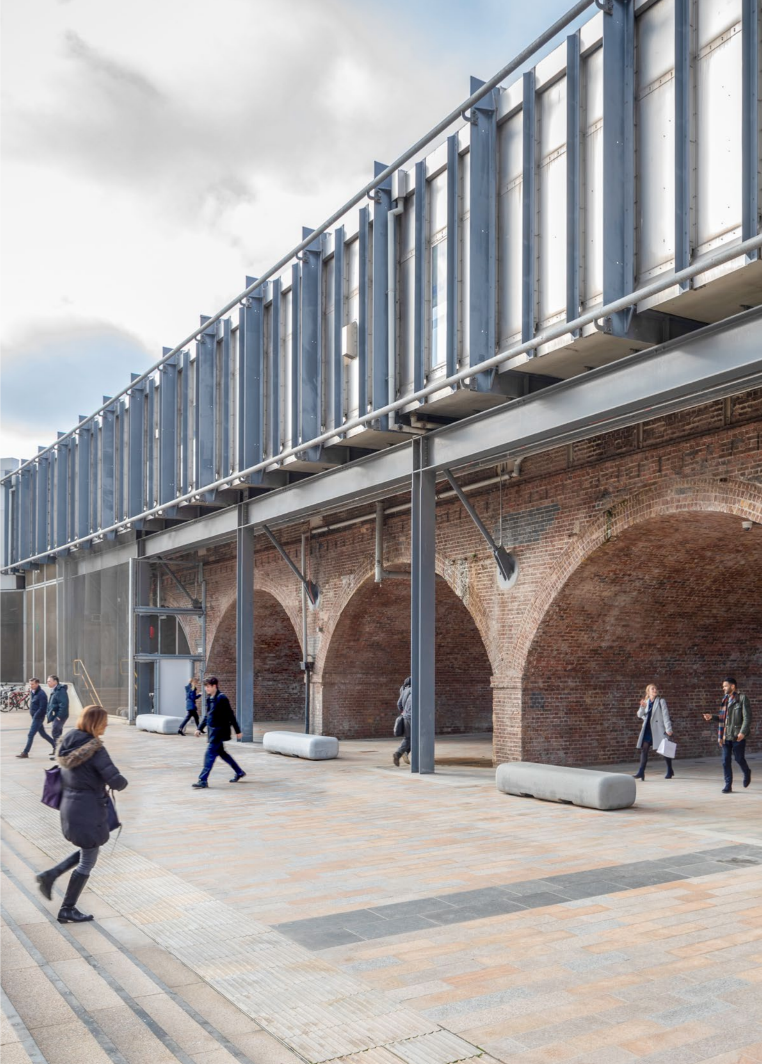
We are creating more retail units in our railway arches
