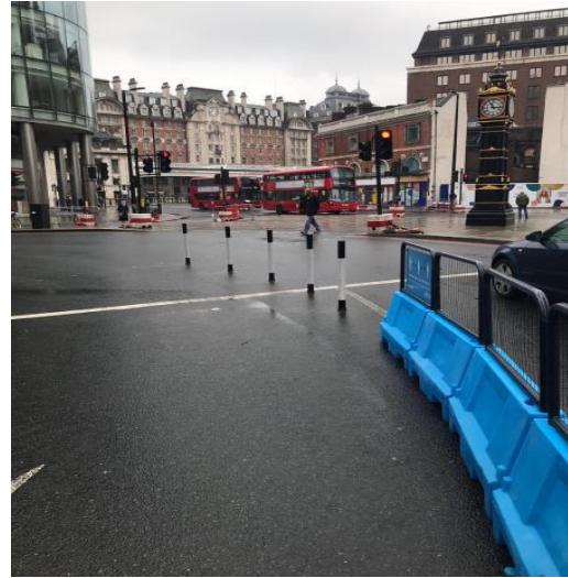
Figure 6: Victoria – Footway widening supporting social distancing at transport hubs and retail locations
