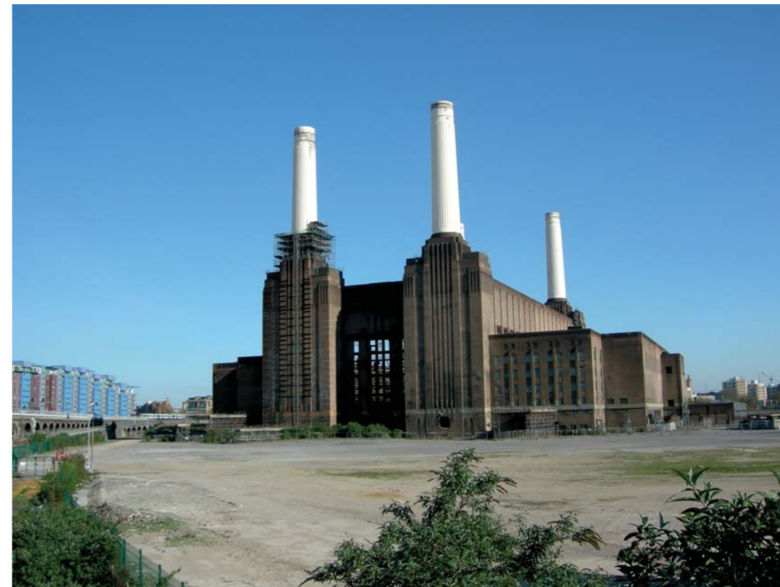
Fig 14 Battersea Power Station looking north-west over Box and Crossover site, taken 16-04-2012
