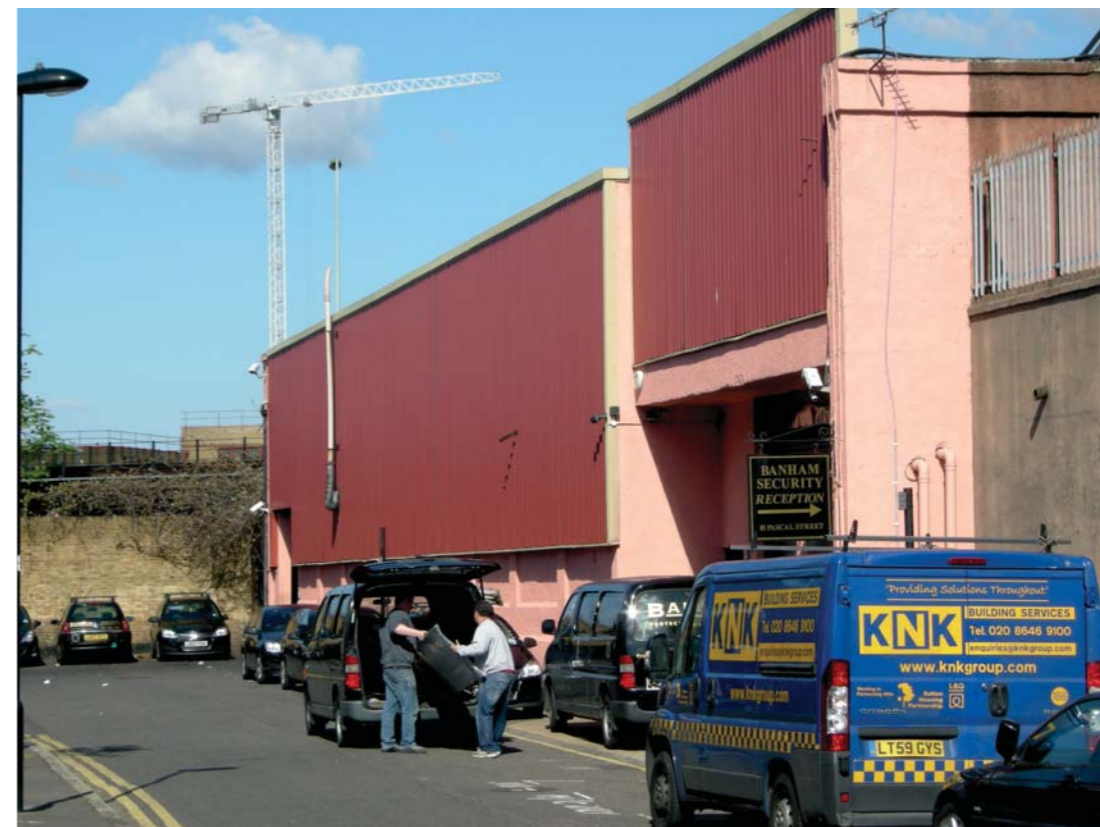
Fig 15 Nine Elms Station Box site on Pascal Street, taken 16-04-2012
