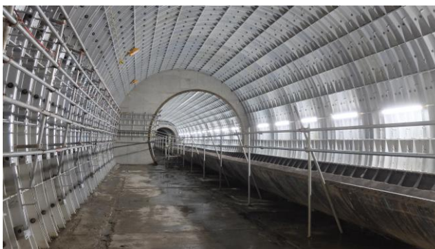
Above – remaining invert tunnel rings to be removed
