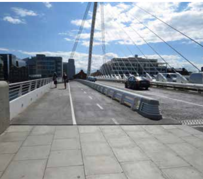
Bi-directional cycle track with separate footway, Samuel Beckett Bridge
