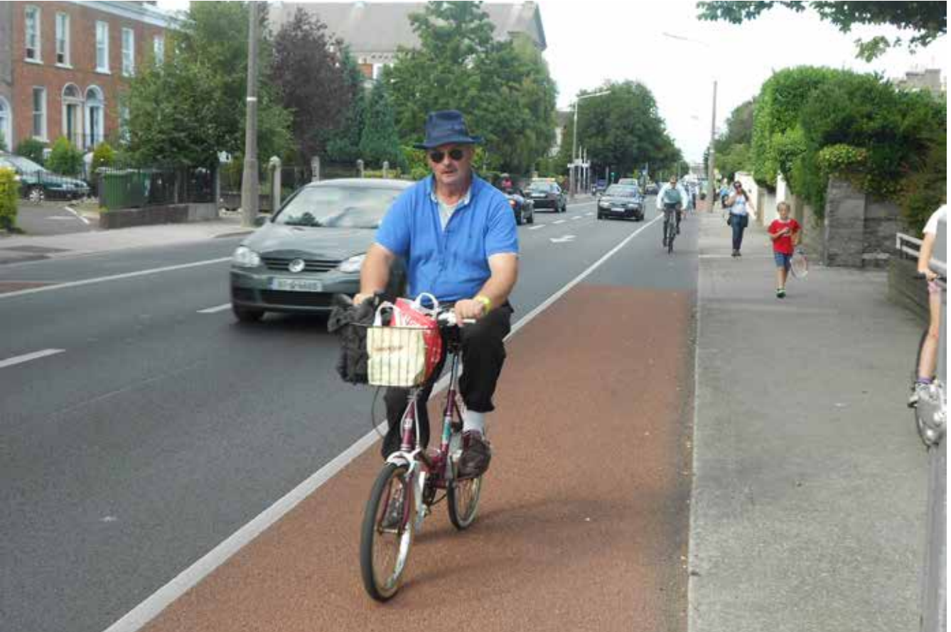
A 2m-wide mandatory on-carriageway cycle lane
