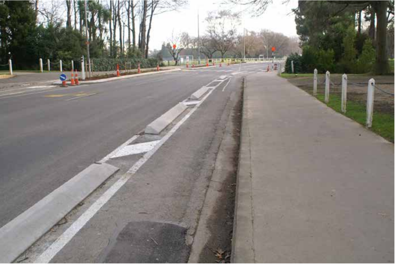
Light segregation on Ilam Road
