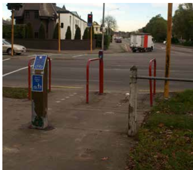
Loops are double to enhance detection and near and far side aspects are displayed
