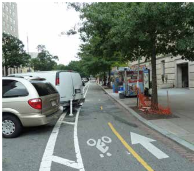
Two-way 'lightly segregated' track with adjacent end-on parking
