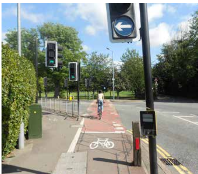
Cycle-only stage at signals across the ring road, leading to a cycle path across green space
