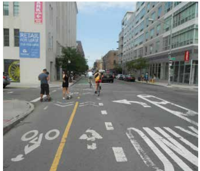
A bi-directional painted lane in Brooklyn
