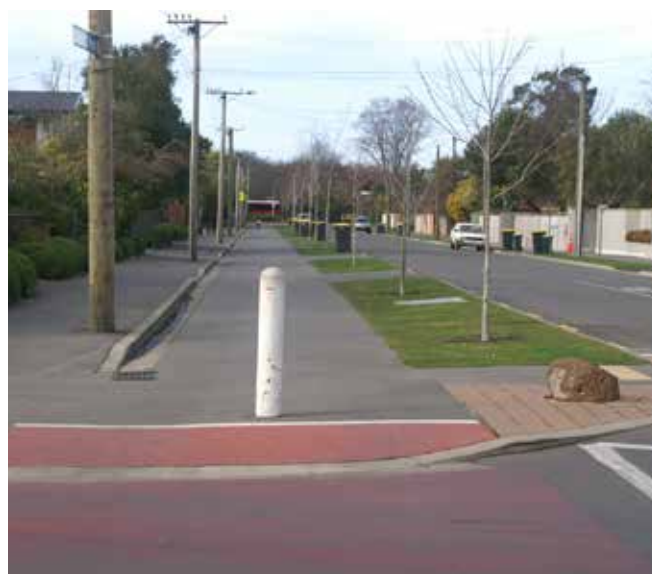
Generously-proportioned cycle route adjacent to road
