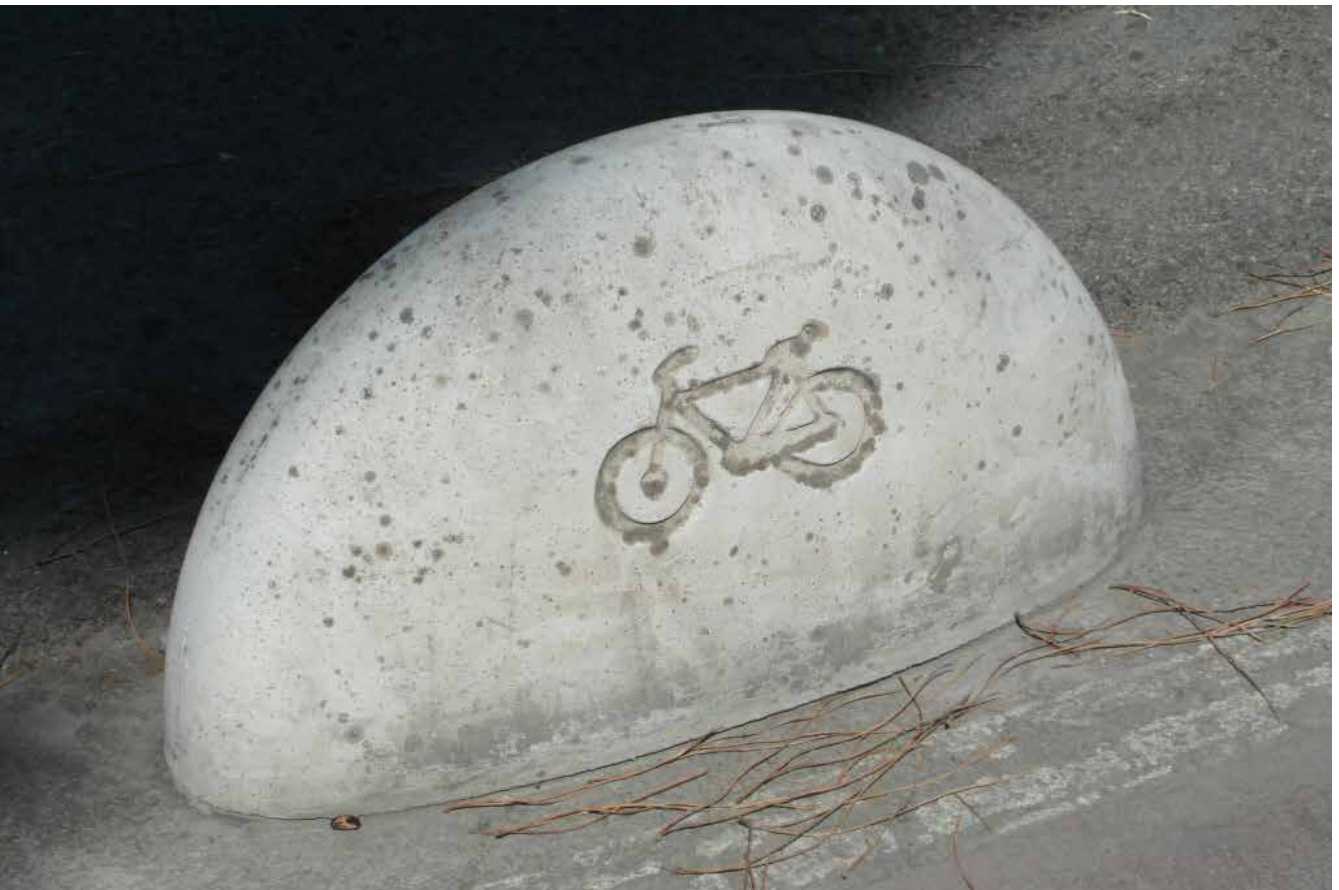
Close-up of a 'Lacasito' - a concrete feature used widely to project cycle lanes (the nickname comes from a Spanish M&M-type sweet)
