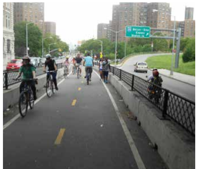
A bi-directional protected bike track in the centre of a major highway
