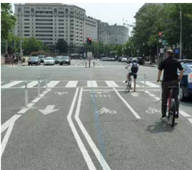
Signalised junction on two-way central track, with separate lanes for ahead and turning movements
