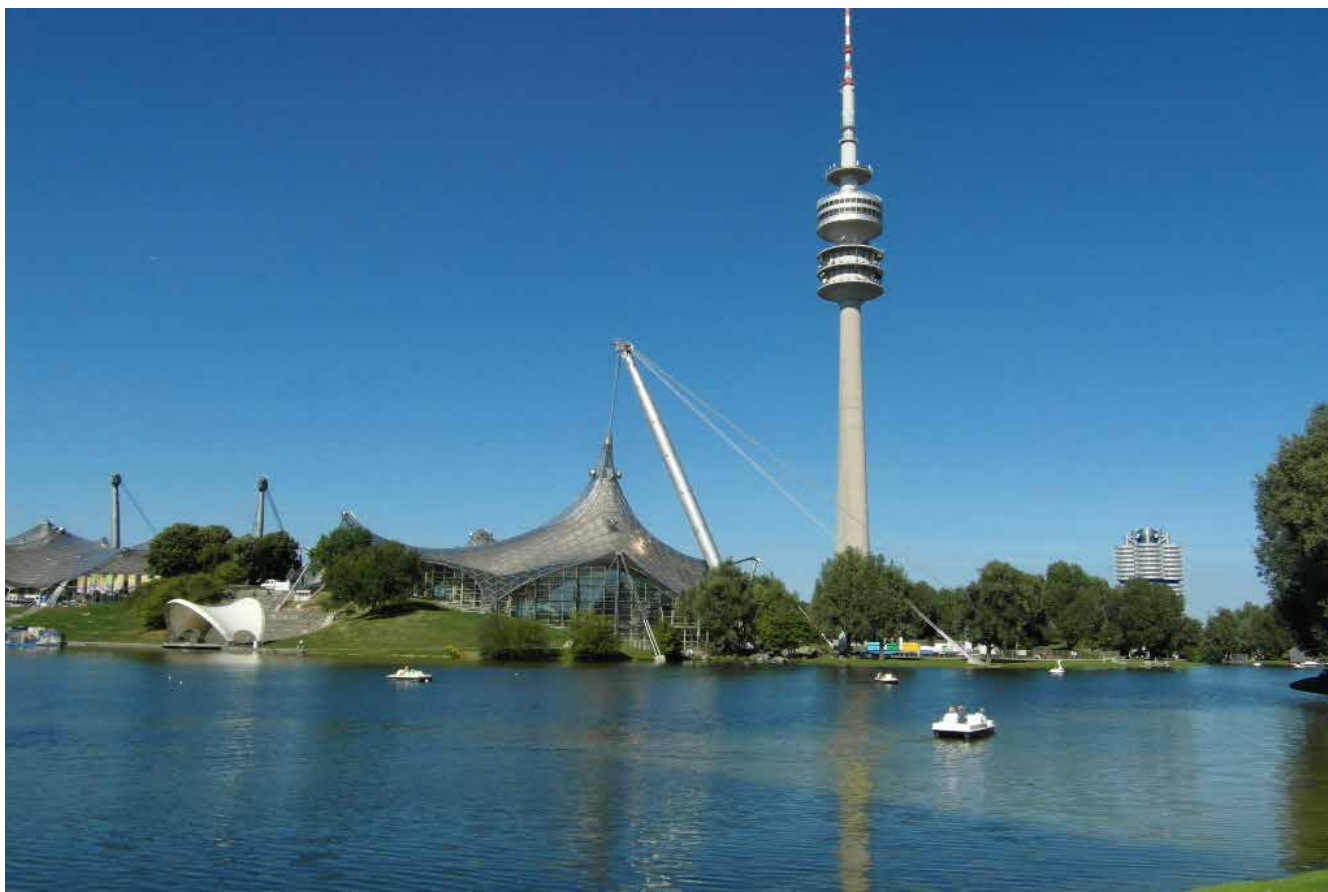
Cycle tracks through the Olympic Park are a great way of getting to and around one of the city's main attractions
