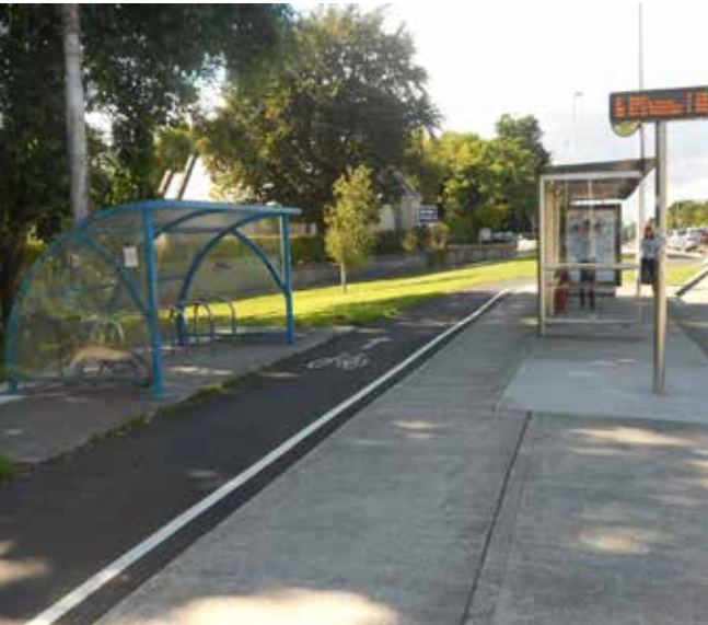
Bus stop bypass and adjacent cycle parking
