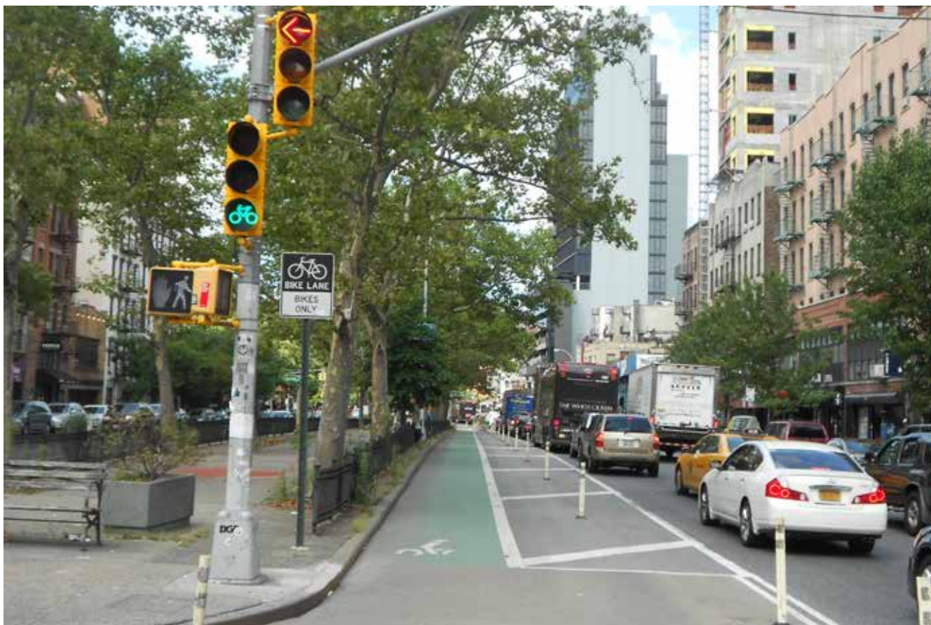
Offside bike track created at low cost with segregation through flexible wands in a wide, painted buffer strip.
