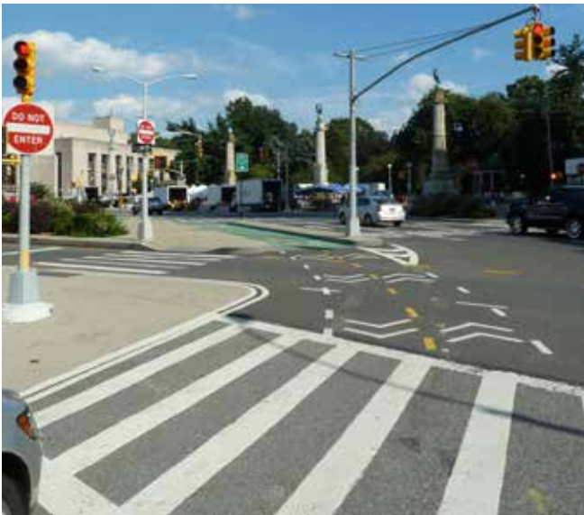
Bi-directional track through a complex junction. Lane markings and 'sharrows' (shared use arrows) help to waymark
