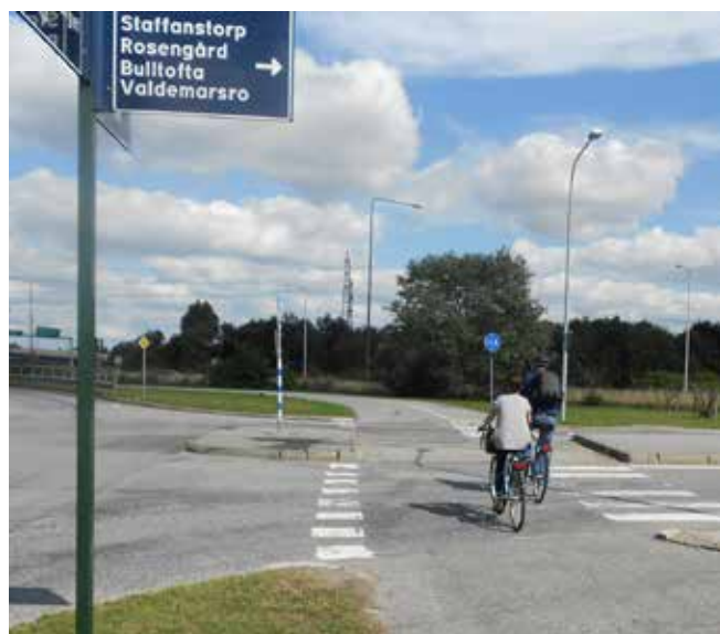
Suburban bi-directional track, again with priority over the side road and with parallel pedestrian crossing
