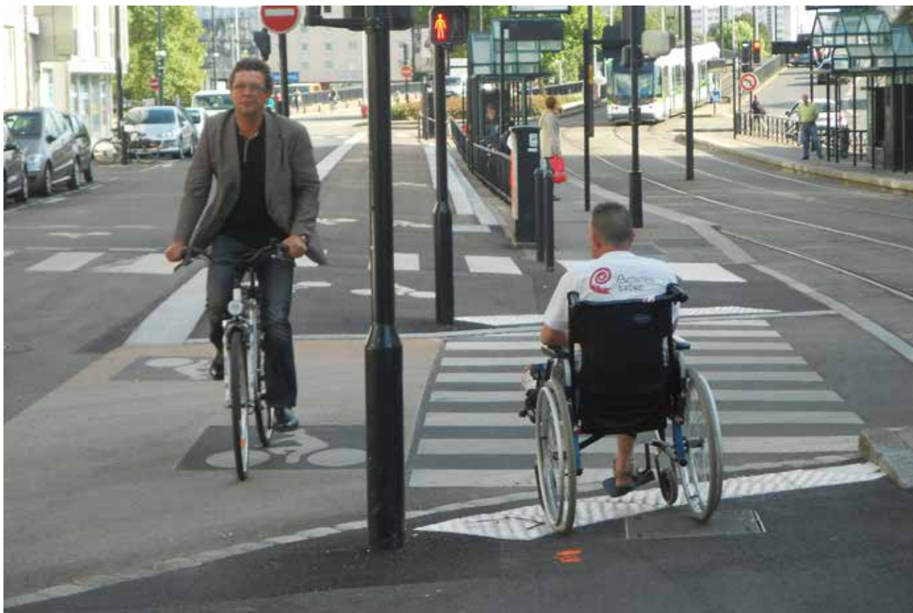
The southern section of the Cours des 50 Otages - parallel cycle and pedestrian crossings over a central reservation gap, next to a tram stop.
