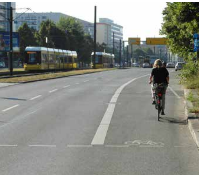
Mandatory cycle lane on a dual carriageway - with dedicated tram zone in the centre
