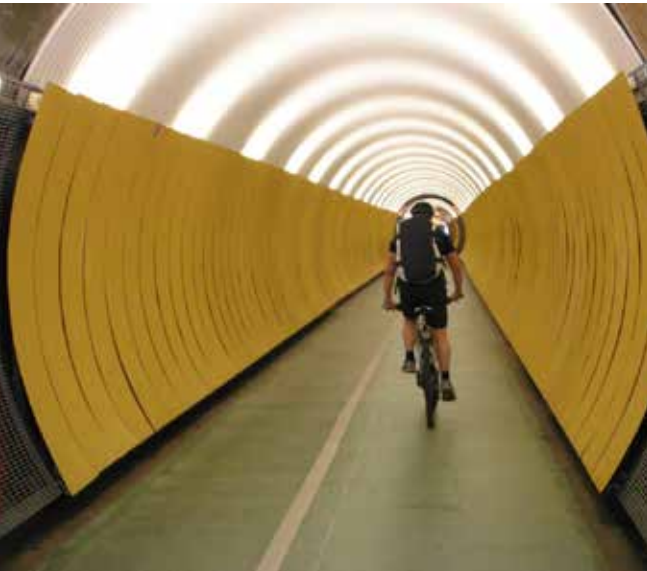
This pedestrian and cycle tunnel in the city centre allows people to avoid a steep ridge.
