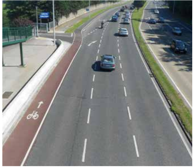
A cycle lane transitioning into a verge cycle track on Stillorgan Road
