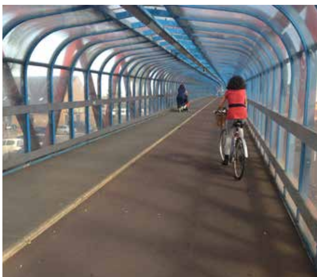
360m long covered pedestrian/cycle bridge across the railway corridor, and important east-west connection
