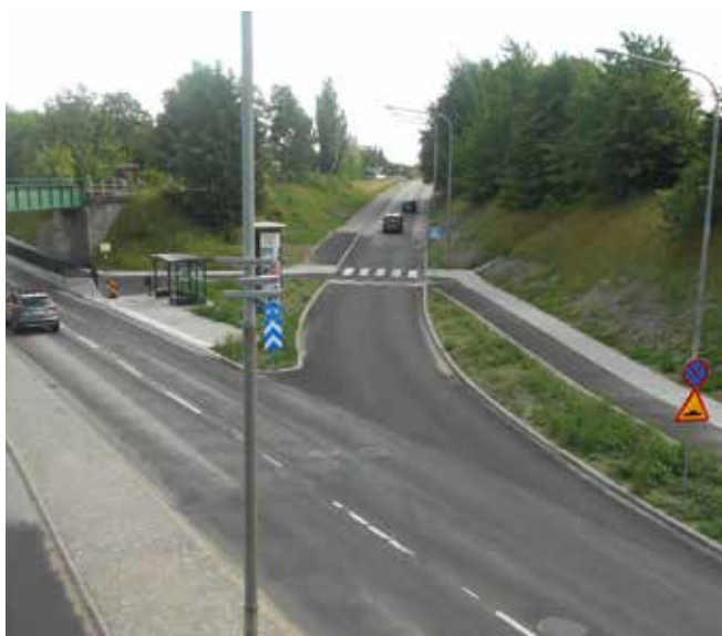
Recent investment in Lund - putting cycle tracks into a large, grade-separated junction
