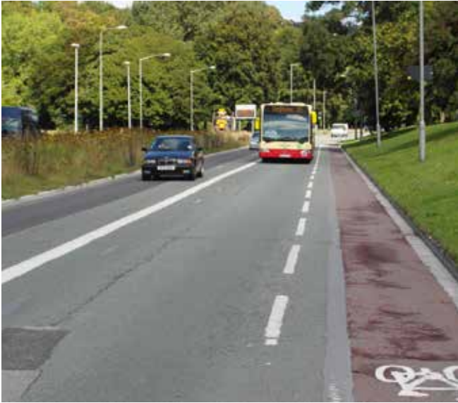
The central reservation on Lewes Road was narrowed to create the wide bus lane + cycle lane arrangement
