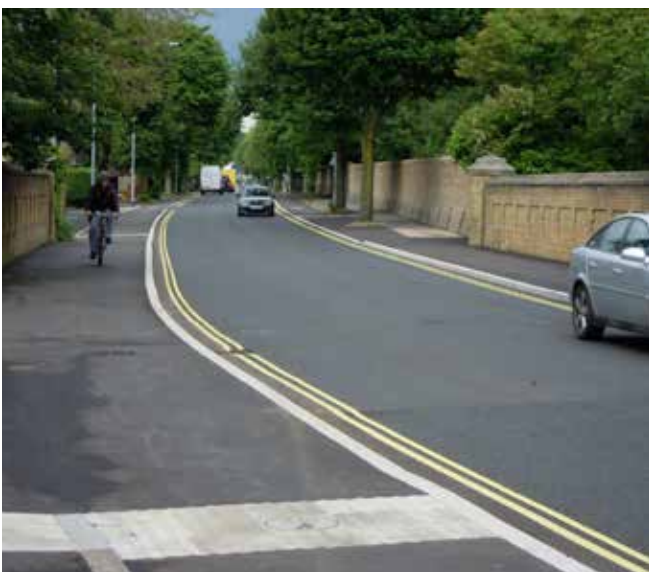
A short section of shared foot/cycle path where Old Shoreham Road narrows to cross a railway bridge
