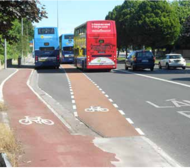
The existing network is made up of both lanes and footway level tracks - which sometimes leads to duplication
