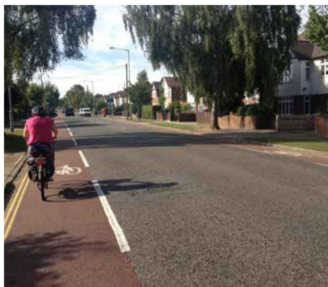
On Gilbert Road, cycle lanes have been widened and the centre-line marking has been removed
