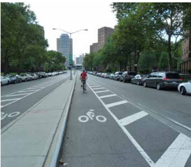
An offside cycle lane with wide, painted buffer strip. Placing the lane here avoids conflict with buses and parked cars
