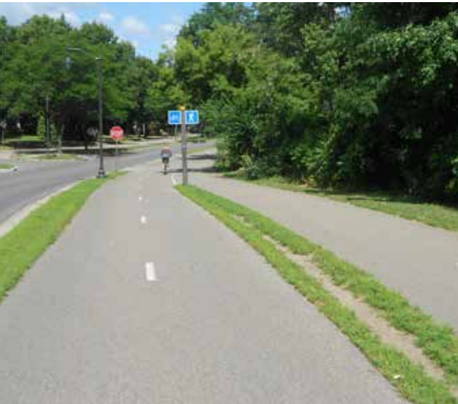
Typical greenway at the side of the road, with separate bi-directional cycle track and footway
