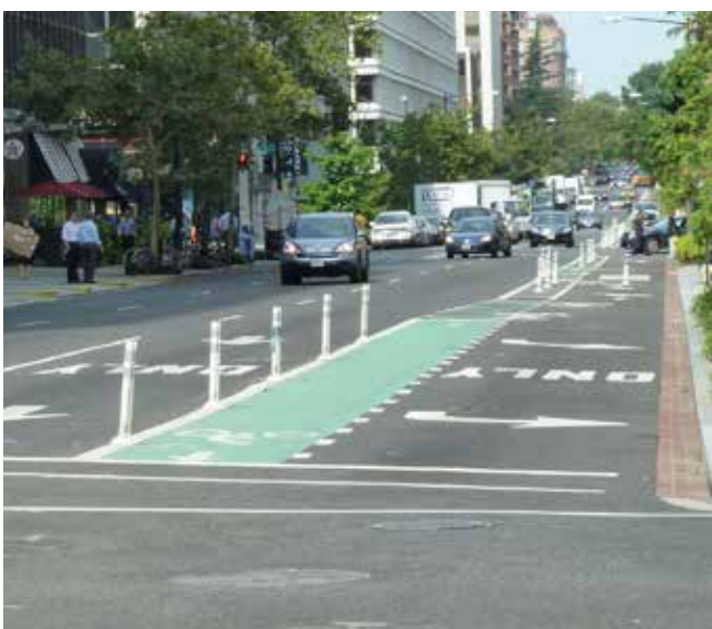
'Mixing Zone' with light segregation to limit area where motor vehicles can move across
