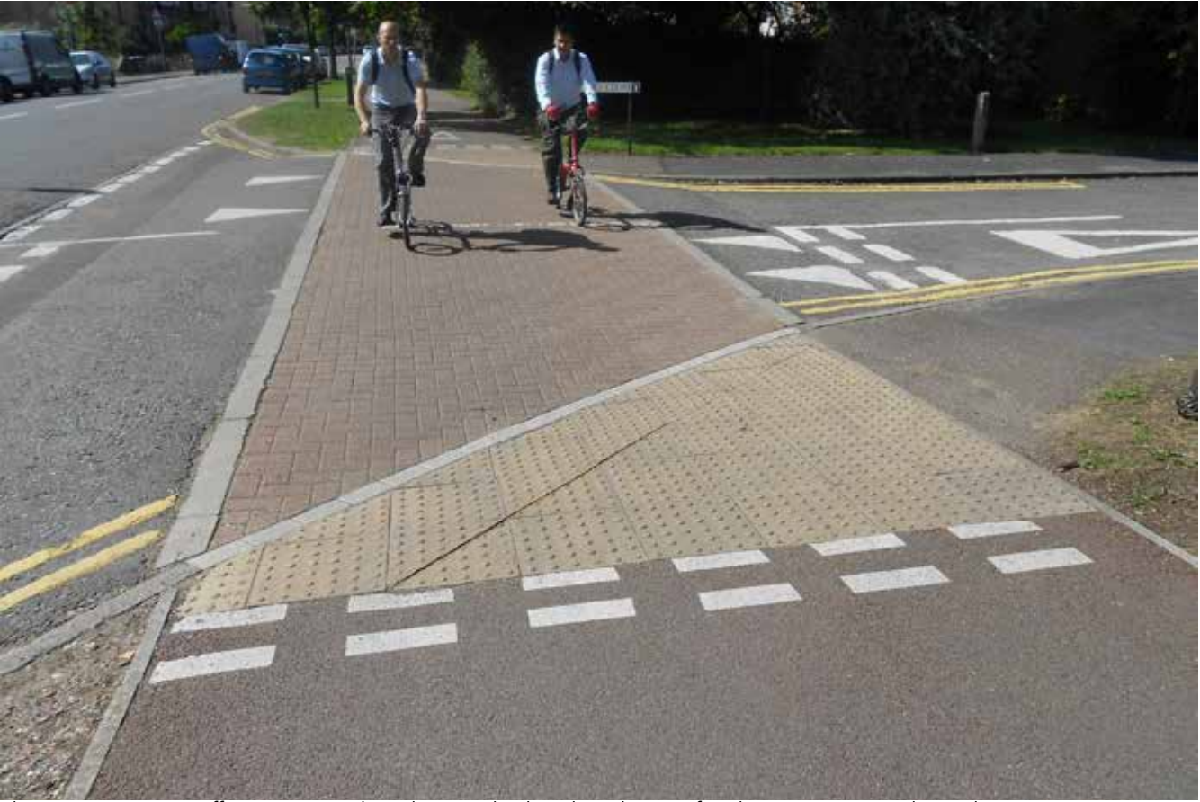
There are numerous off-carriageway shared use paths, but they do not often have priority at side roads
