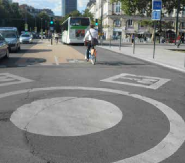
Nantes has many roundabouts and has placed cycle symbols in the circulatory carrieway at some of them
