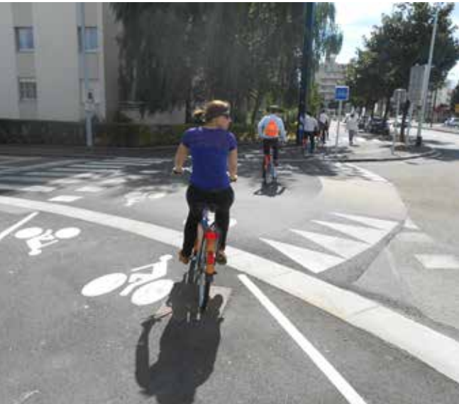
A recent extension to the main bi-directional track across the city - with priority over side streets
