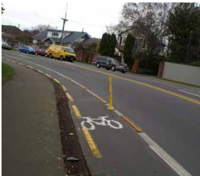
Flexible vertical markers and Riley separators
