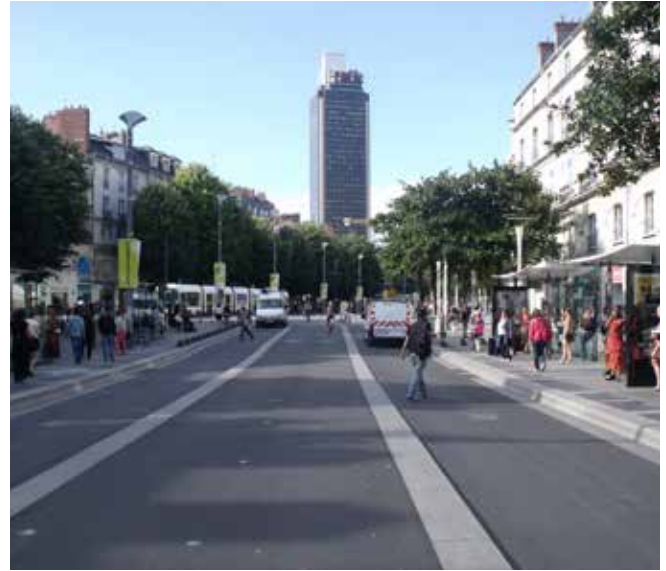
Central, bi-directional track, Cours des 50 Otages; with bus lanes to either side
