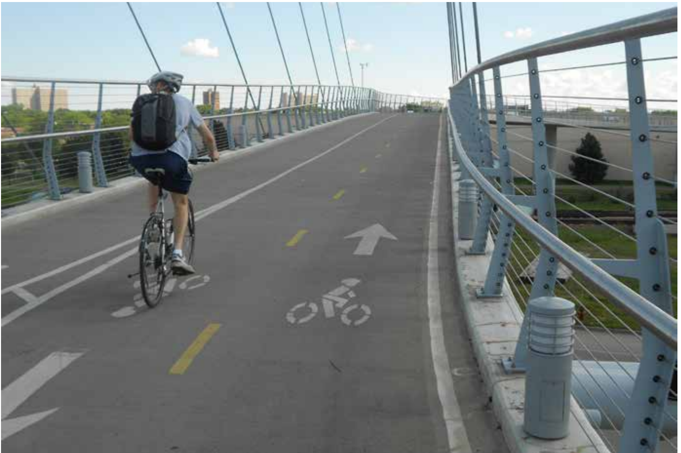
The Martin Olav Sabo bridge, carrying the Midtown Greenway across Hiawatha Avenue (Trunk Highway 55). It is 671m long and is divided into a bi-directional cycle track and a footway
