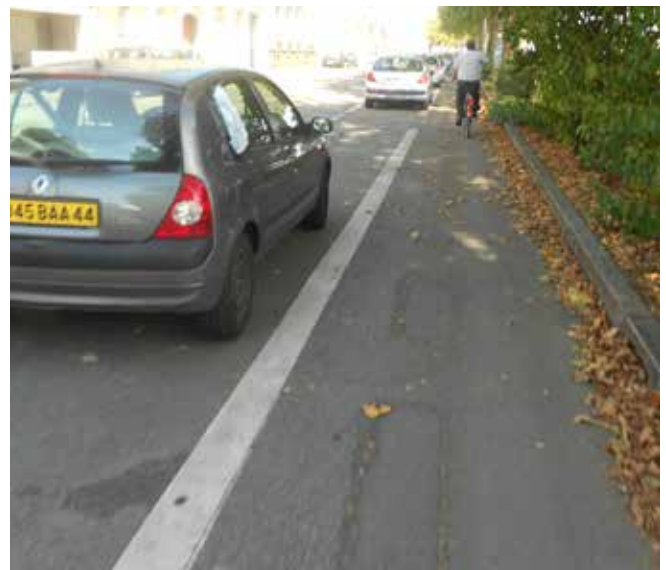
Painted lane with offside car parking
