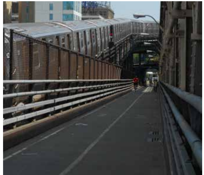
There is cycle provision (of varying quality) across all the major bridges in NYC
