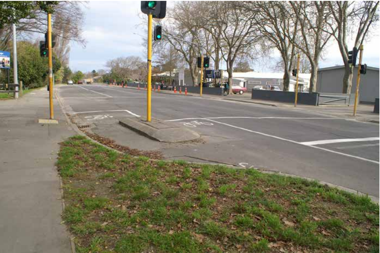
Cycle ahead and right turn movements provided with separate facilities at a signalised junction
