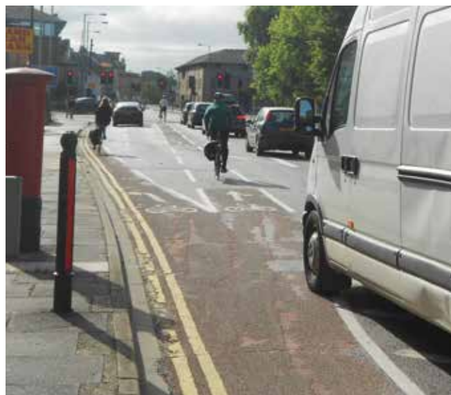
Central cycle lane on approach to traffic signals, to separate ahead cyclists from left-turning traffic at the stop-line.
