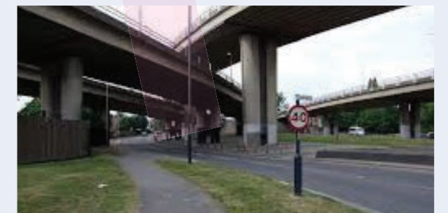
New pedestrian and cycle crossings, and fewer delays to traffic and buses
