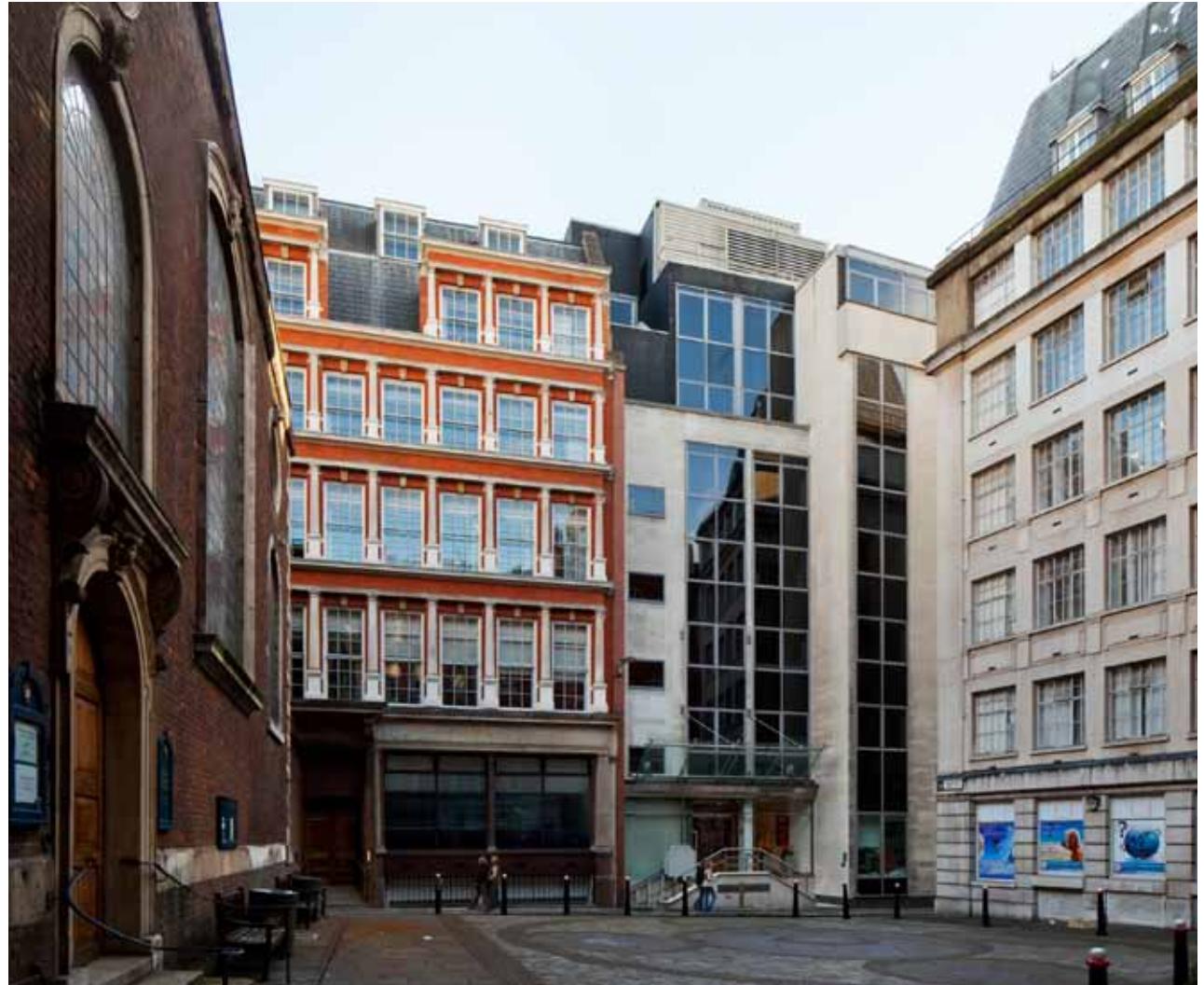
View of the Whole Block Site from Abchurch Yard, with the Grade I listed St Mary Abchurch (left) providing important townscape character
