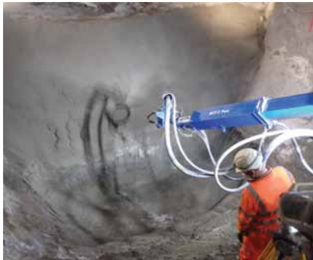
Application of sprayed concrete lining to a tunnel
