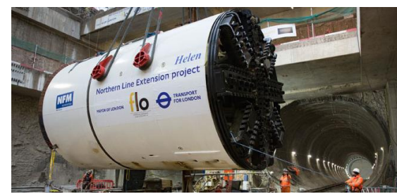
Northern Line Extension Restarted works at Battersea and Nine Elms
