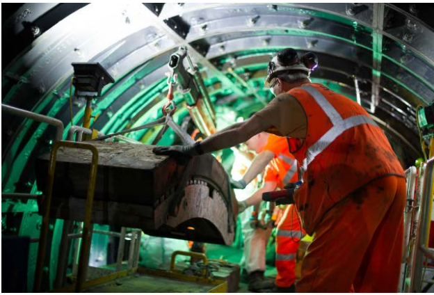
Tunnel ring segment being lowered on cradle
