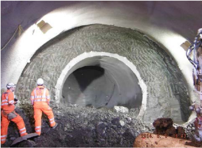
Bond Street station excavation works
