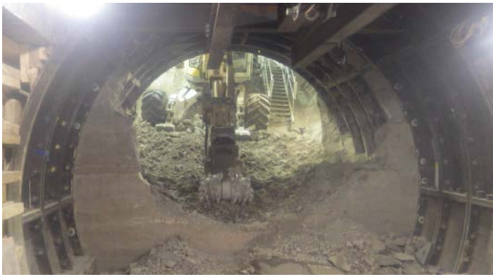
Victoria station excavation breakthrough into the concourse
