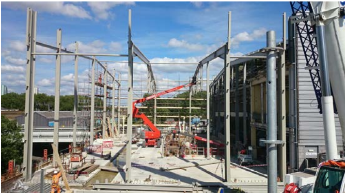
New Cross Gate Depot steelwork
