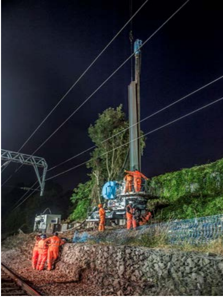
Piling at West Hampstead
