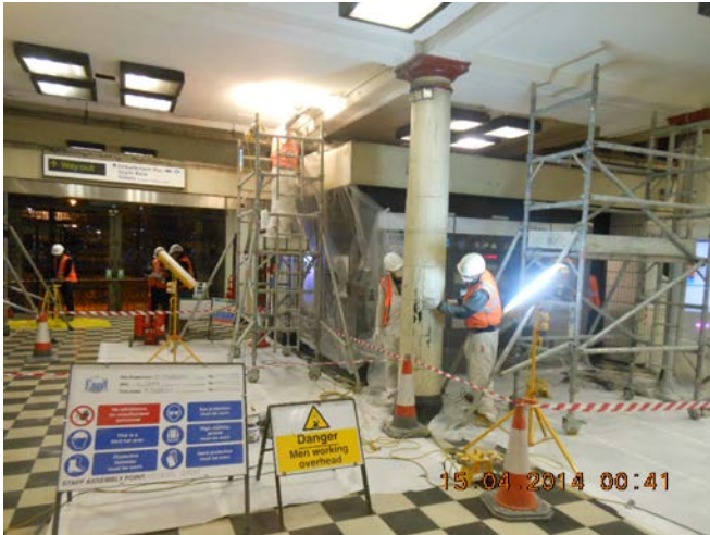
Improvement works at Embankment to freshen up the ticket hall
