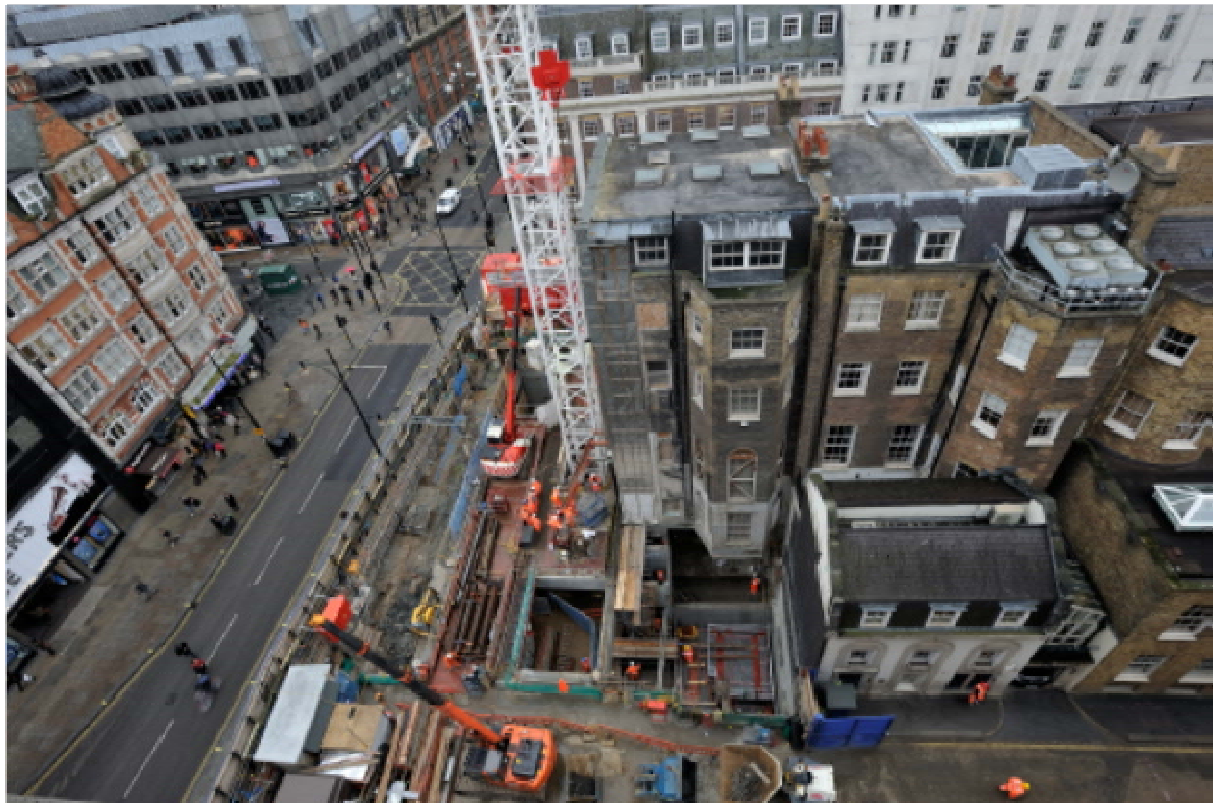
View over site
