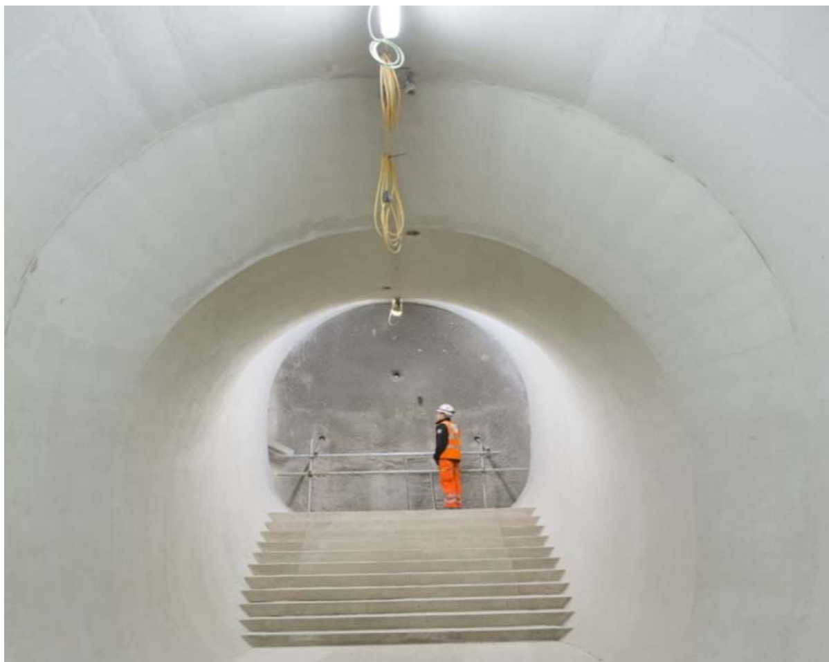
Northern line passage linking through to Crossrail
