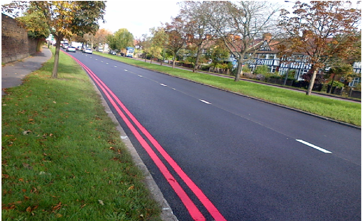
Completed resurfacing works on the A406 North Circular Road / Gunnersbury Avenue
