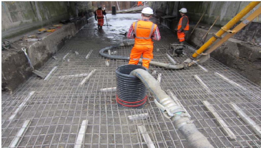
Installation of reinforcement bars before concrete pour
