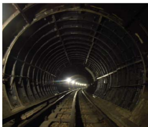
Post installation of 15 rings
