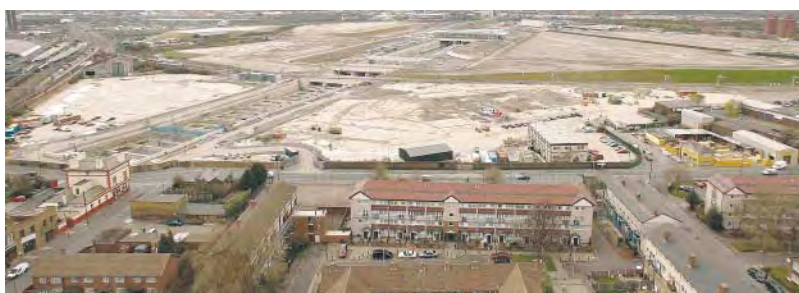
Work is under way at the Olympic Park.
