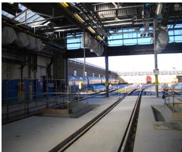
Ruislip depot shed conversion completed
