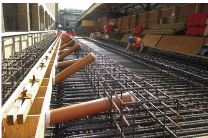
Platform track slab laying at Wimbledon station
