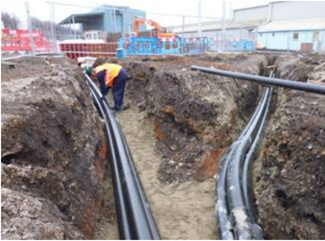
Cable-laying at Neasden depot.
