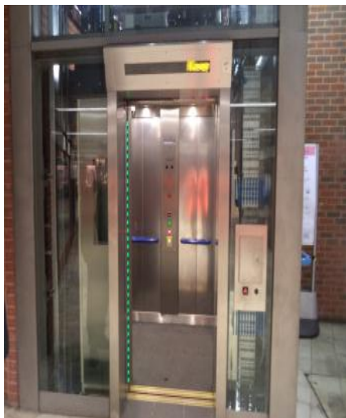
Completed lift at West Ham station
