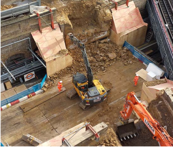
Whitechapel Station Winthrop St bridge removal
