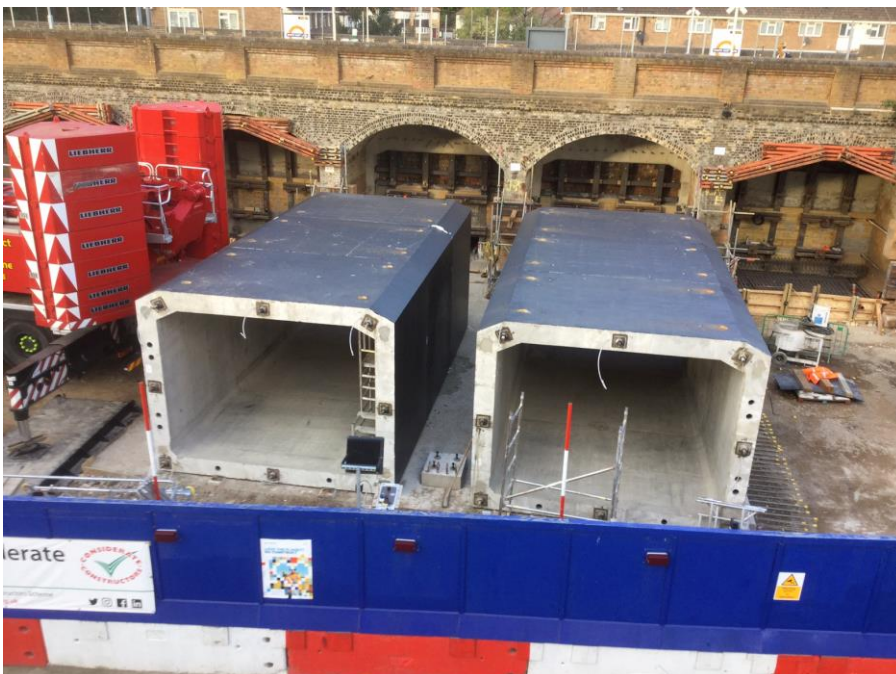
Figure 5 New White Hart Lane pre-cast passenger passageways
