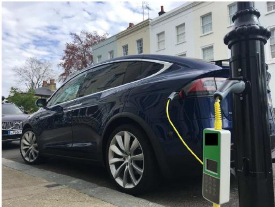
Figure 2. Lighting column charge point. (Image: RB of Kensington and Chelsea)
