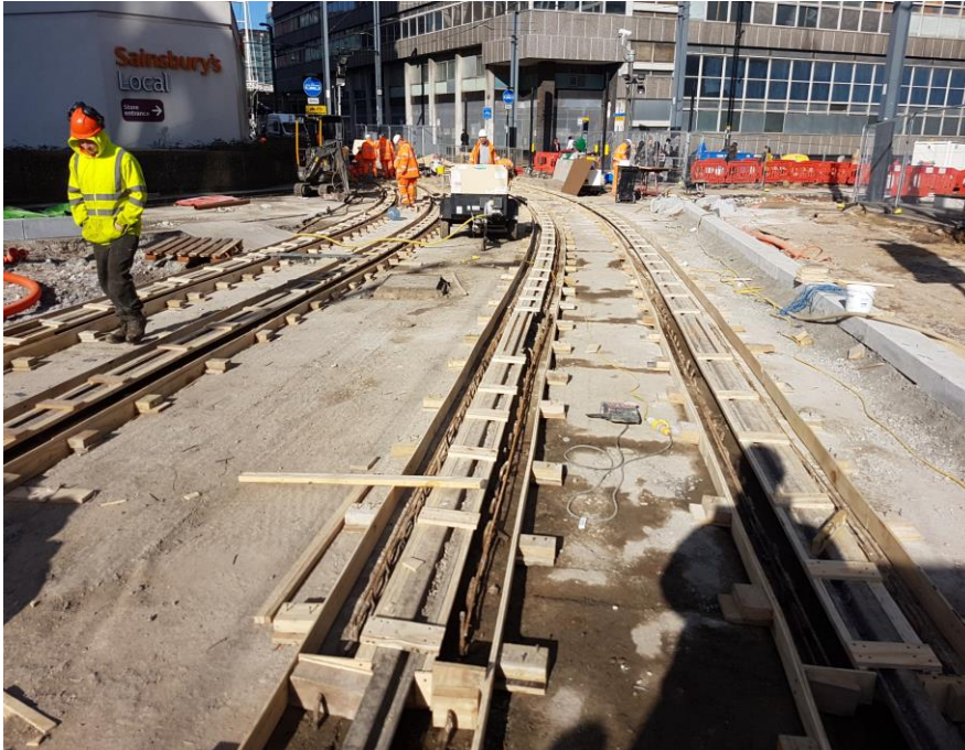
Figure 3 Renewal of the tram track sections in Croydon town centre
