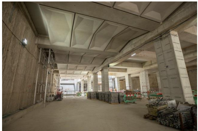
Photo 3 (below): The architectural coffered ceiling in the station ticket hall.
