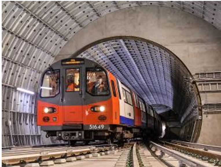
Photo 1: One of the new step plate junctions connecting the NLE tunnels to the rest of the Northern Line.
