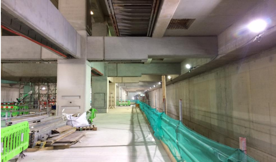
Photo 8: The installation of the pre-cast platform sections is progressing to programme.
