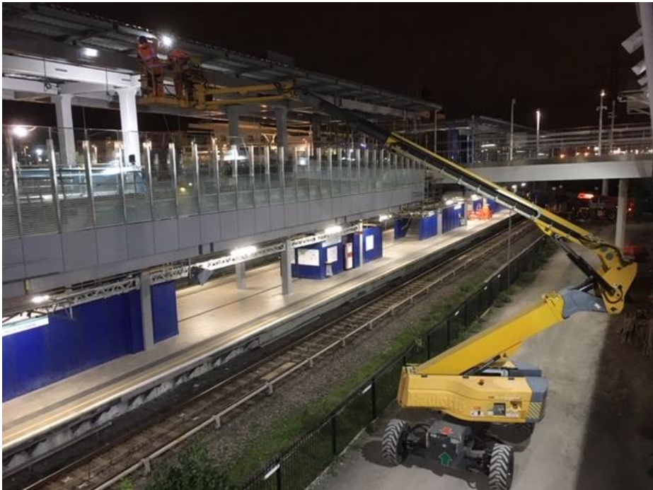
Figure 4 Construction of Custom House station capacity upgrade
