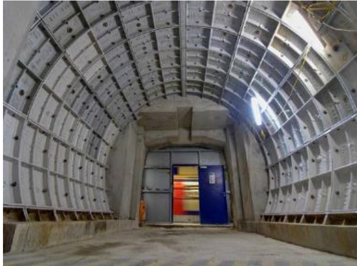
Photo 7: One of the new cross passages
