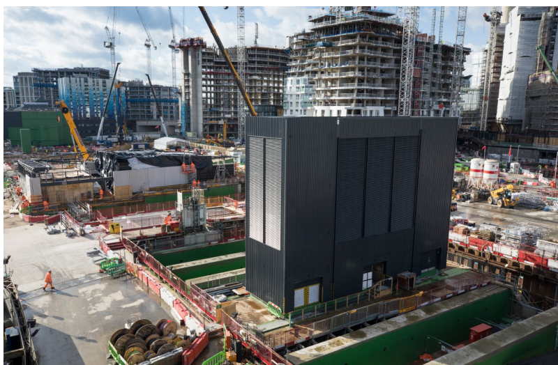
Fig. 1 Eastern ventilation shaft cladding complete
