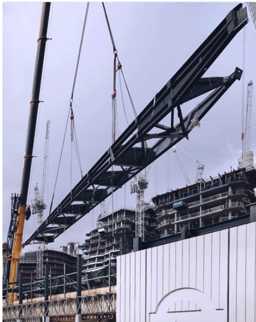
Fig. 3 Steelwork at the entrance to the station
