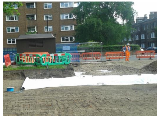
5) Topsoil strip
