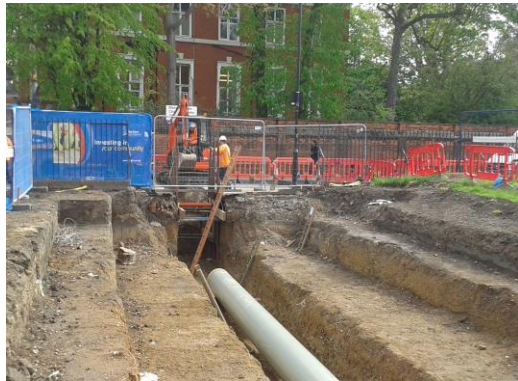
4) Laying New Gas main
