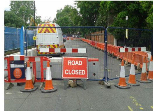
3) Closing of Road for Gas Diversion
