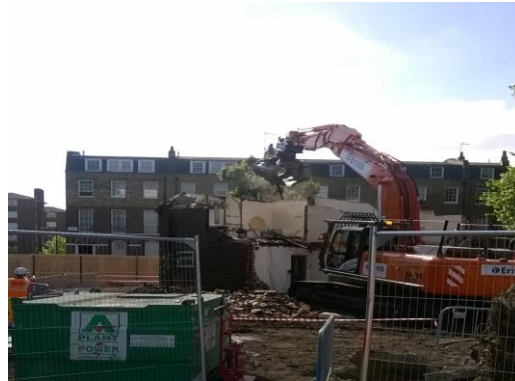
2) Demolition of Lodge
