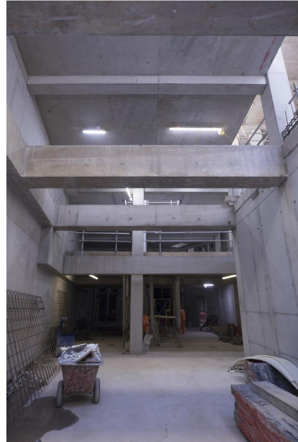
Construction of the basement structure
