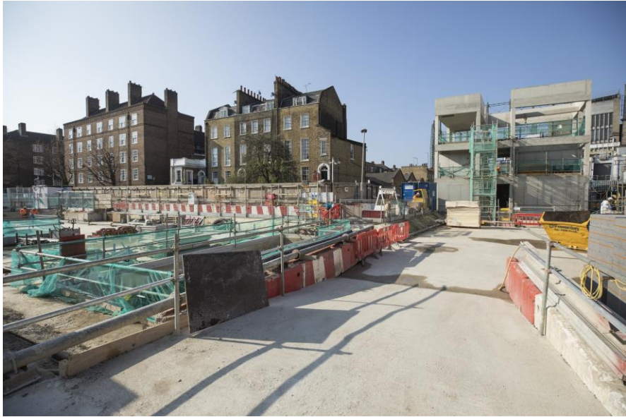
Construction of the headhouse structure
