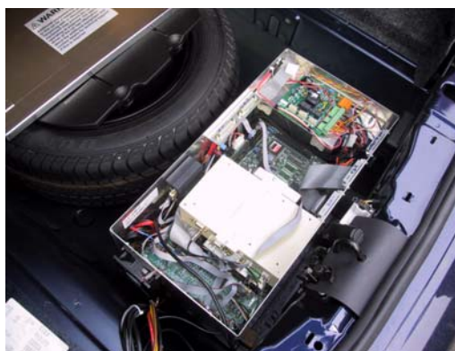
Figure 13: The main ISA equipment installed under the luggage storage area
