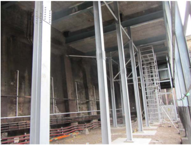
Floor strengthening steelwork as Farringdon
