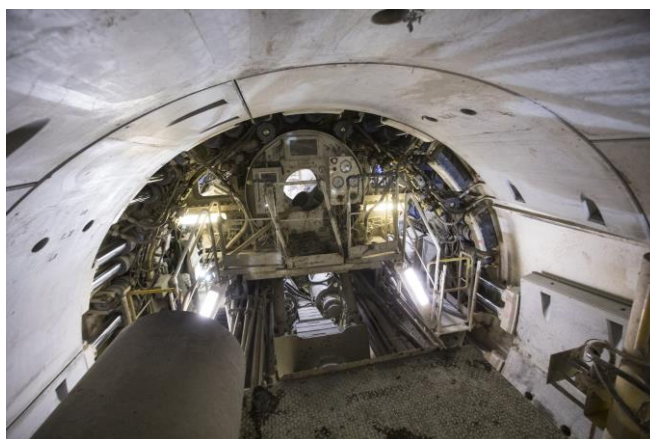
Above – inside the Tunnel Boring Machine
