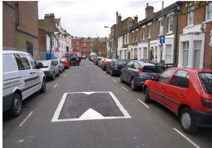
Figure 5: Speed cushions on a one way street
