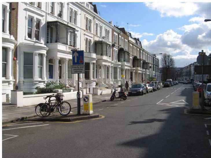
Figure 7: A Chicane with priority over oncoming traffic
