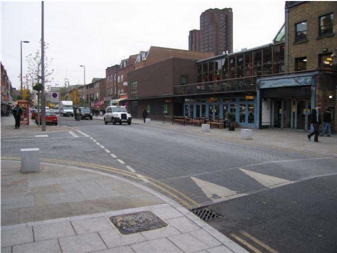
Figure 9: A raised junction
