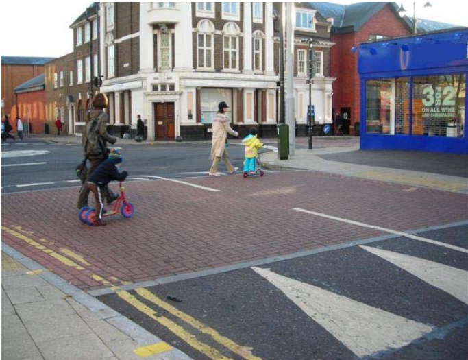
Figure 8: A side raised entry treatment
