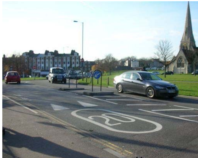
Figure 12: A raised informal crossing point and pedestrian refuge with 20 mph roundel painted on the carriageway
