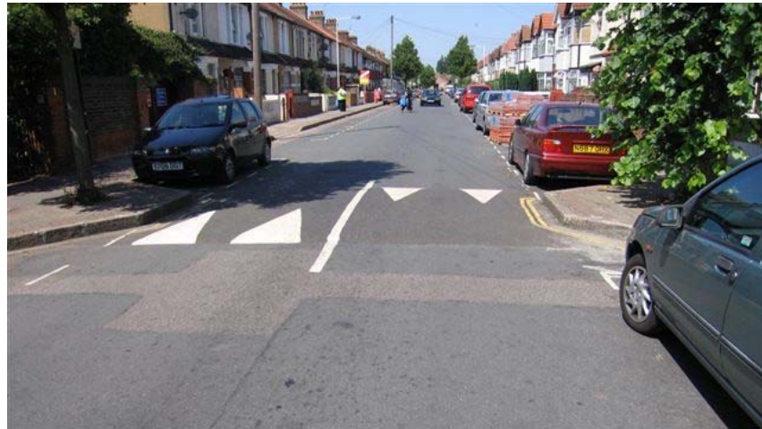
Figure 3: Speed hump on a narrowed section of road
