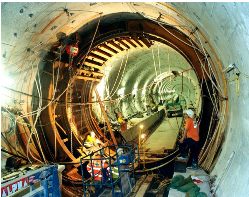
Cross Passage Construction CTRL C320
