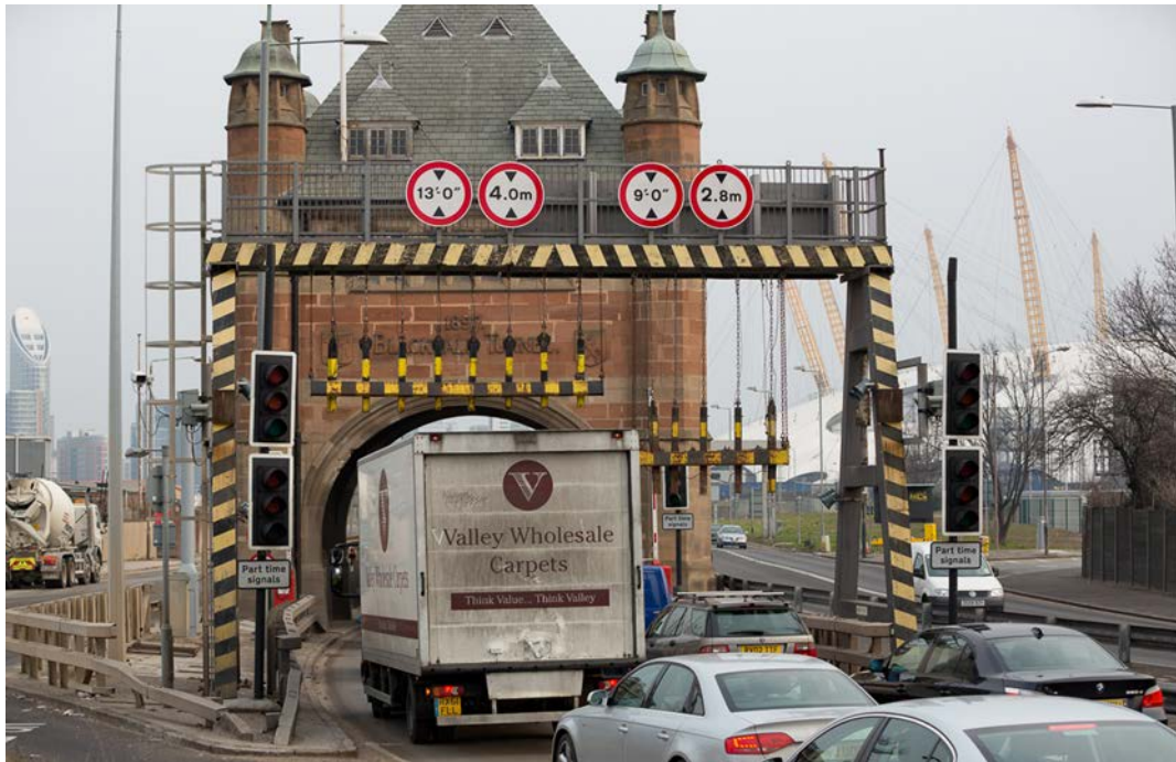
Figure 2-17: Blackwall Tunnel northbound bore height restrictions
