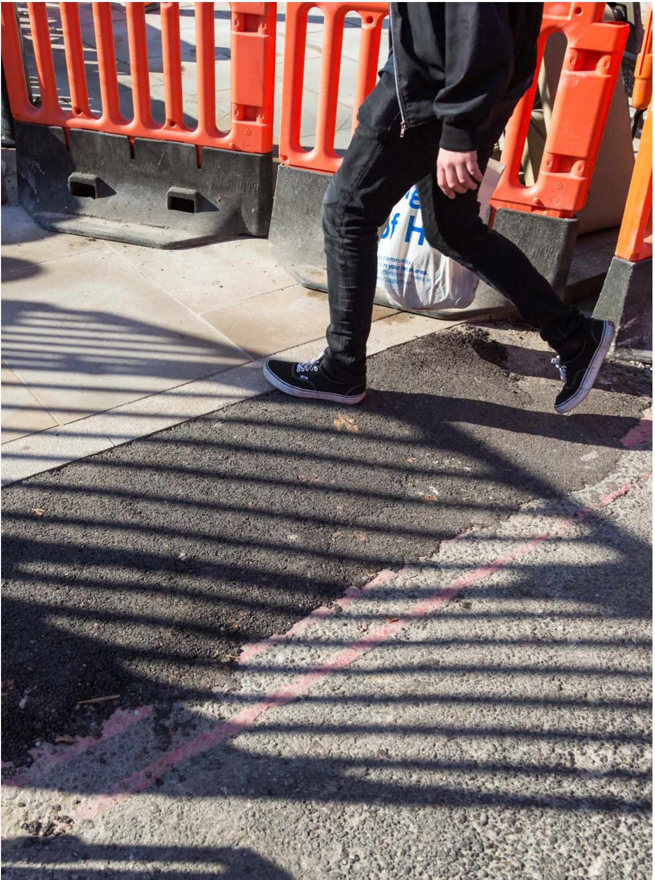
Temporary tarmac footway
