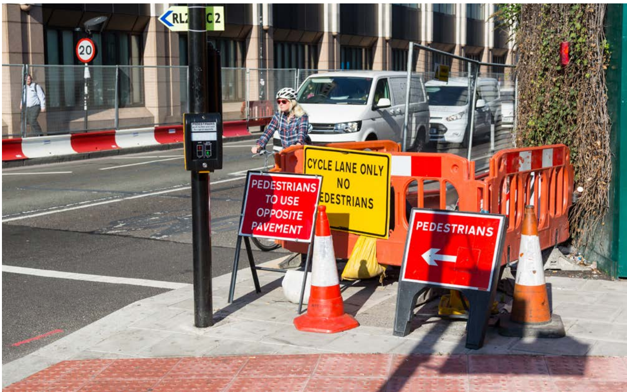
Bad practice: confusing and non-compliant signs, with non-standard wording and sign clutter
