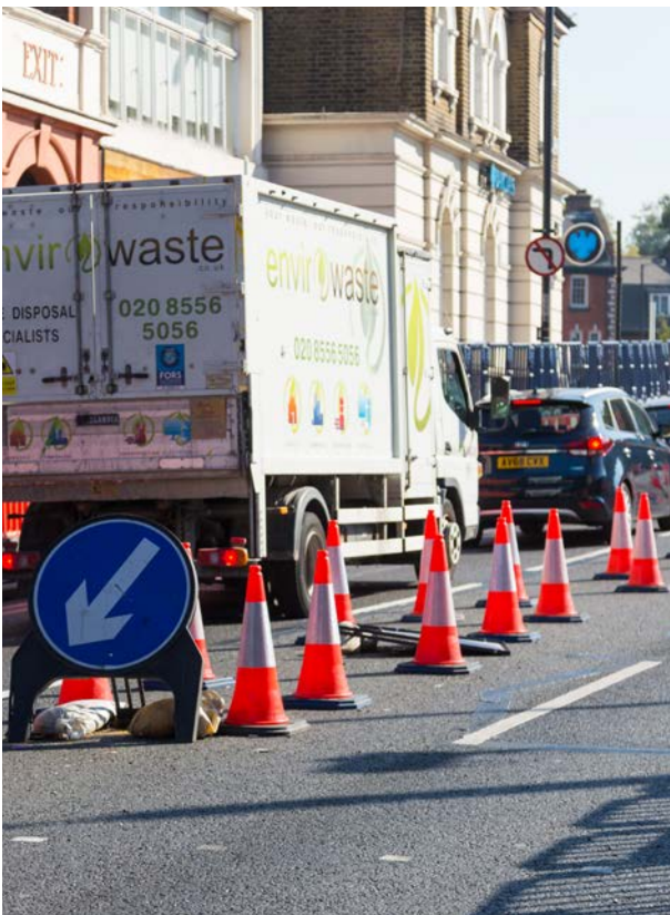
Well-maintained traffic cones keep a site safe and routes clearly defined
