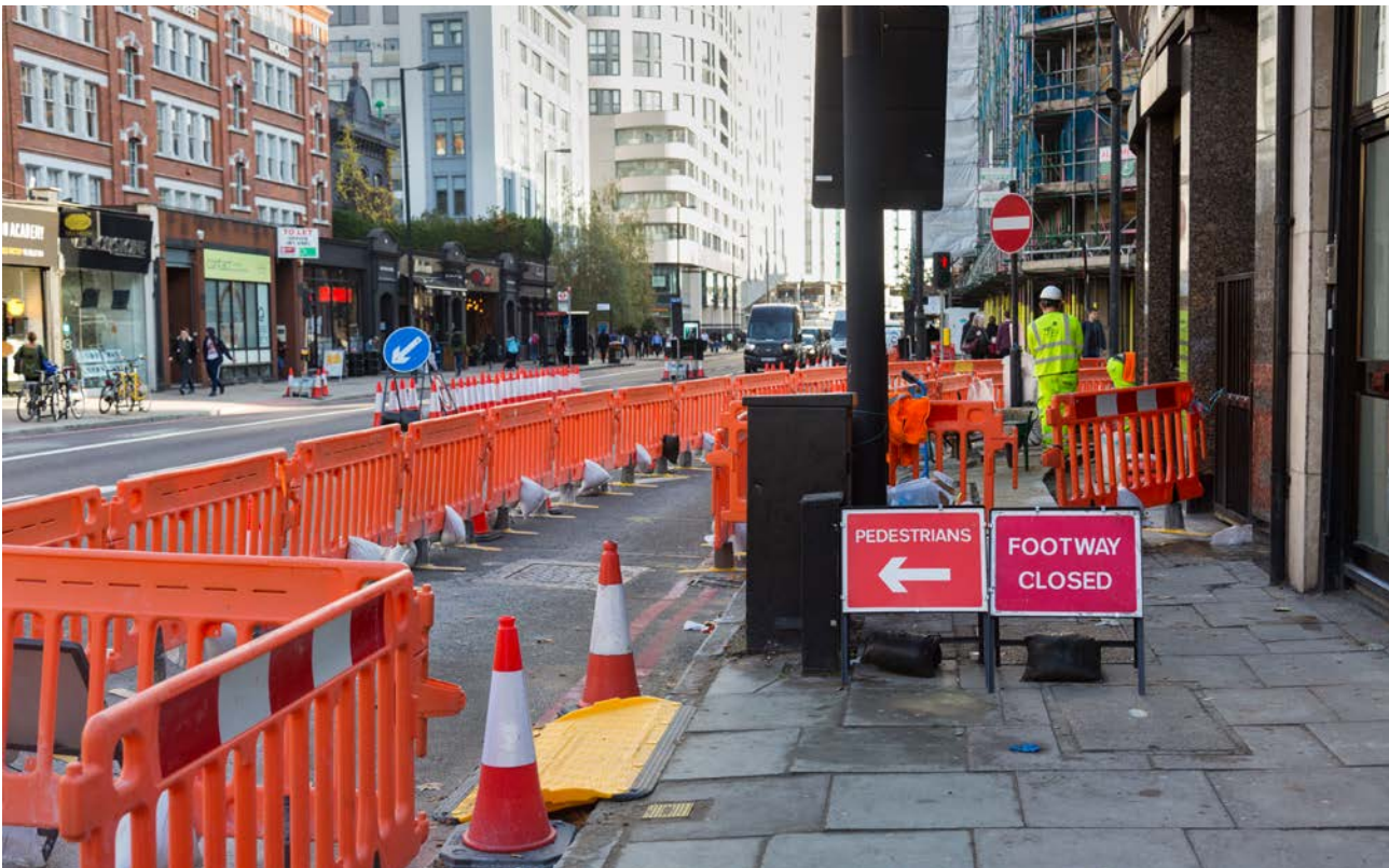
Closed footway with temporary walkway in carriageway
