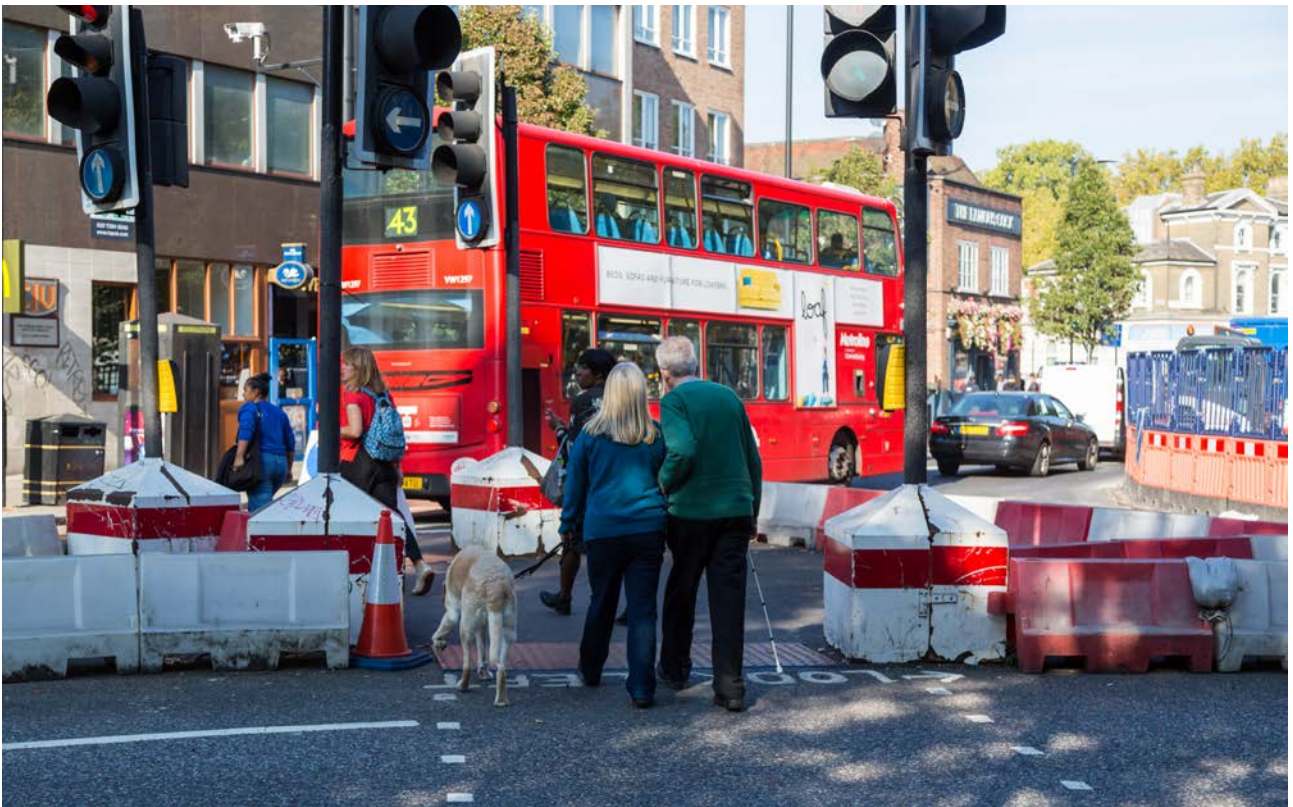
Site-specific risk assessments must also consider the needs of visually impaired and disabled people
