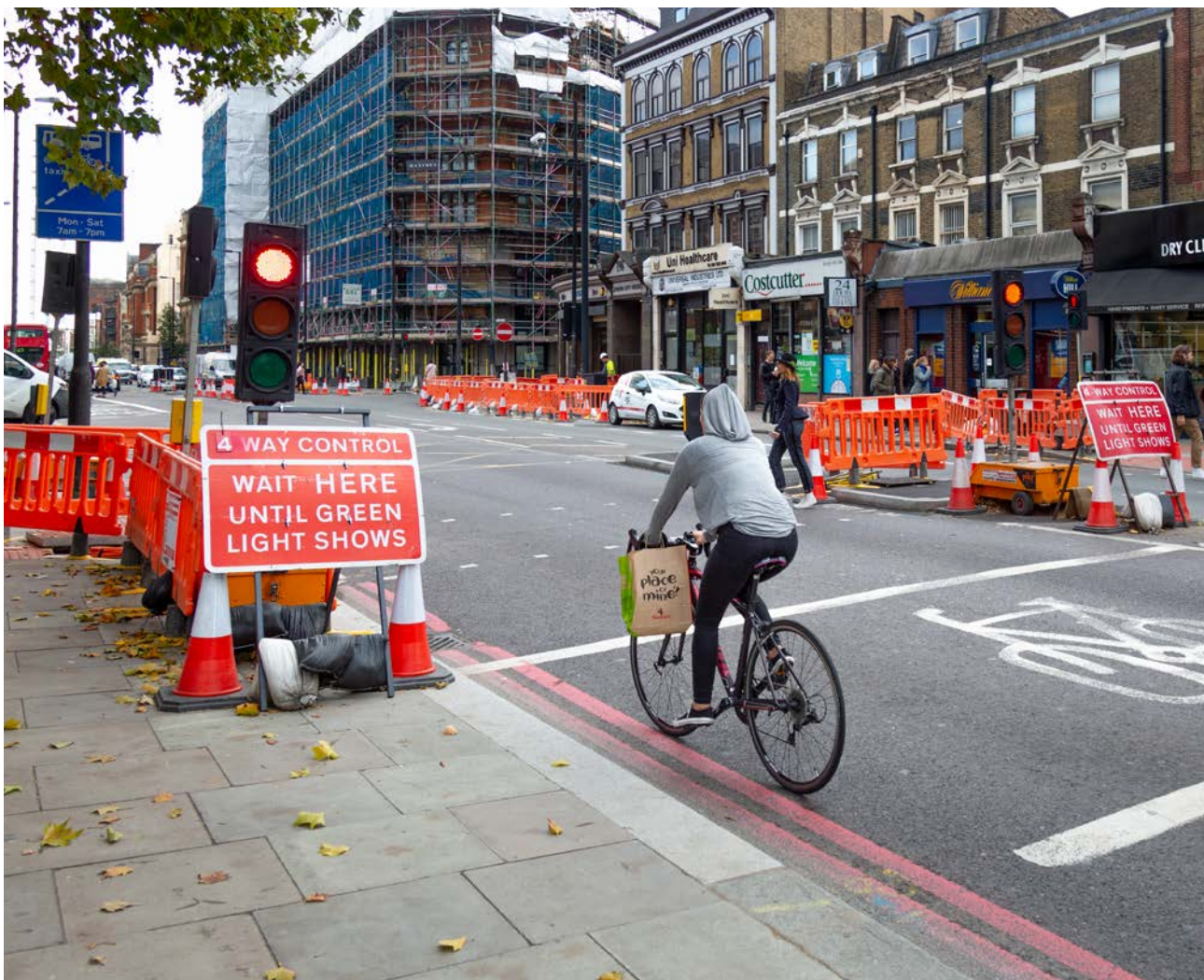
Ensure signal heads and 'Wait here' signs do not prevent cyclists using advanced stop lines
