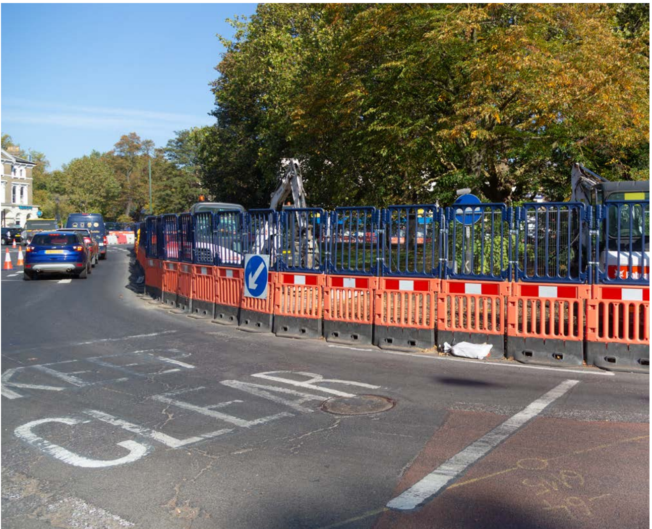
Well-maintained and appropriate barrier
