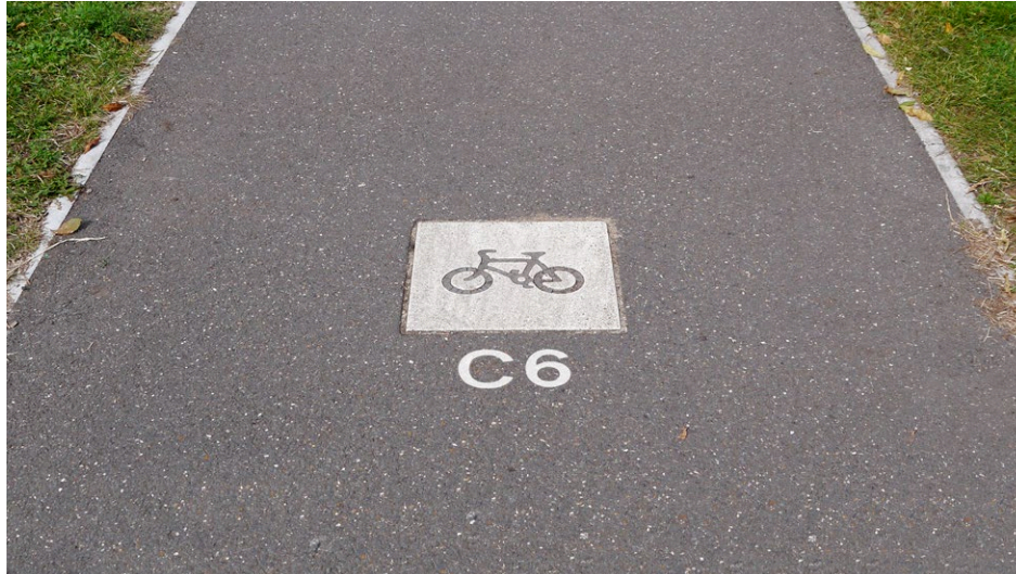
Existing cycle only path with C route number reassurance where required.
