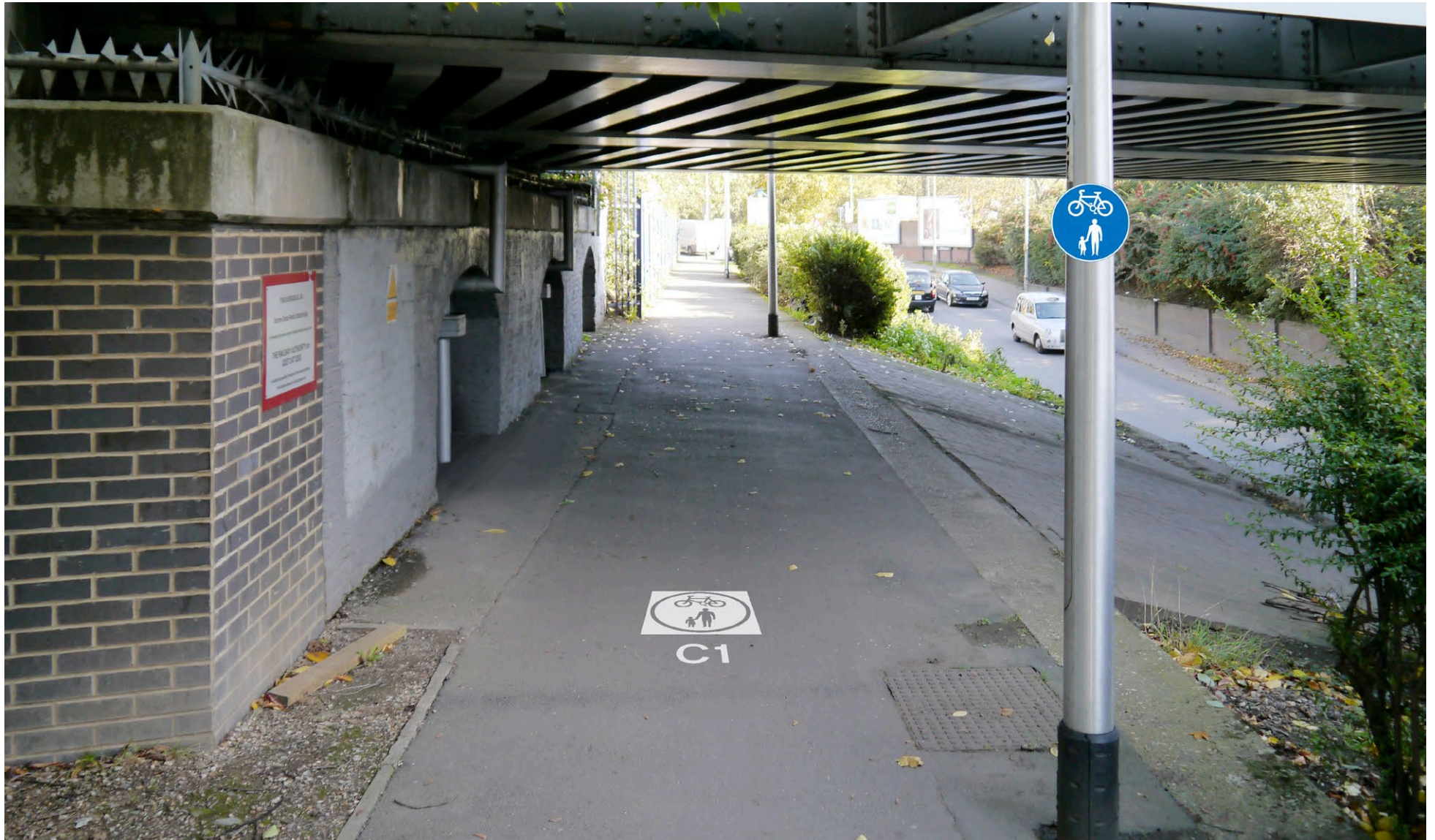
Shared use footway, mid link – shared use sign to diagram 956, with optional context-specific surface marking showing route number, for continuity
