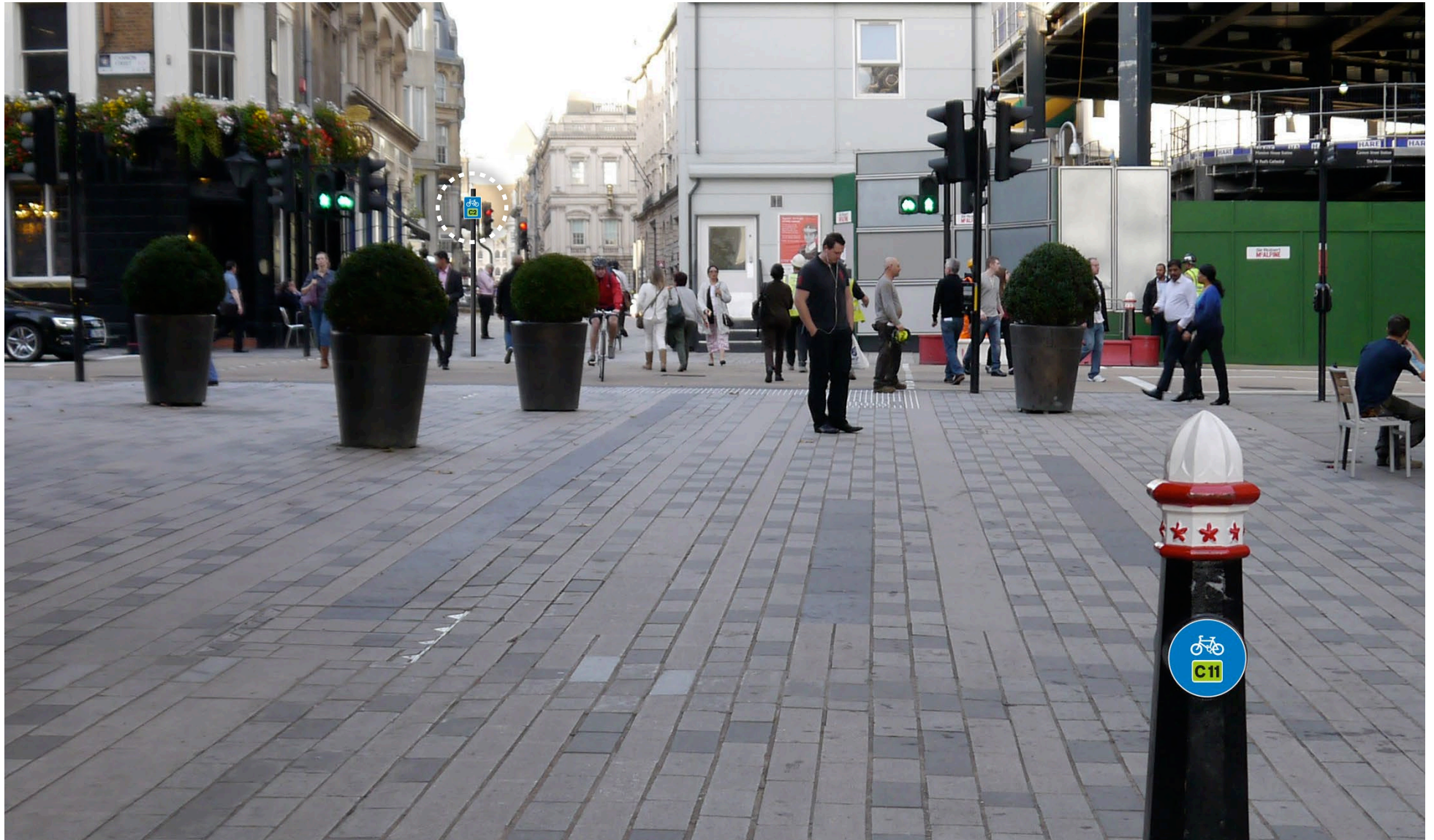
Public highway, crossing (toucan) – see through confirmatory.
