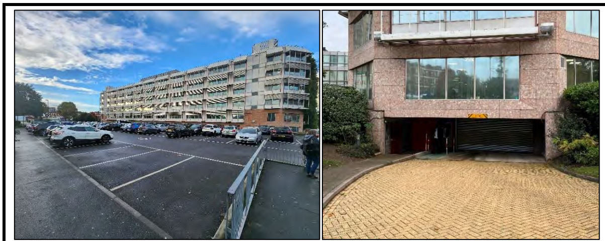
Figure 34 Existing Laurence House’s ground floor car park and basement access
